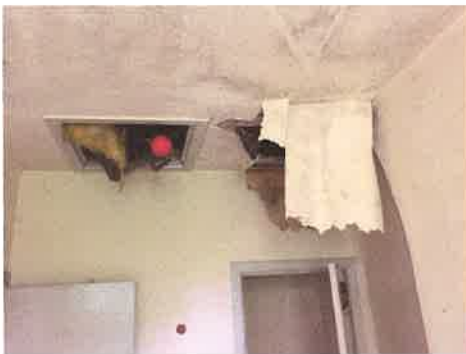
Fig 6 Water Tank Unit2 blocking hatch Replace
