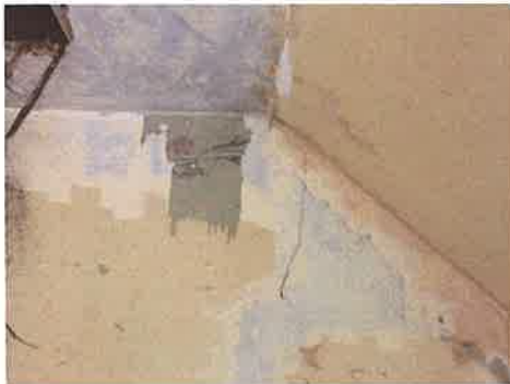
Fig 15 Roof spread to Unit 3 Install ties
