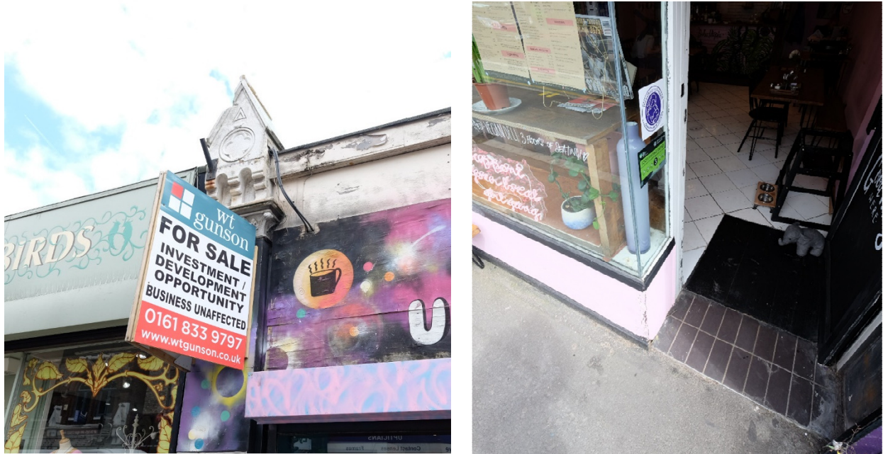
Fig 5 & 6: Stone console ahead stone pilaster, recessed entrance to no. 485
