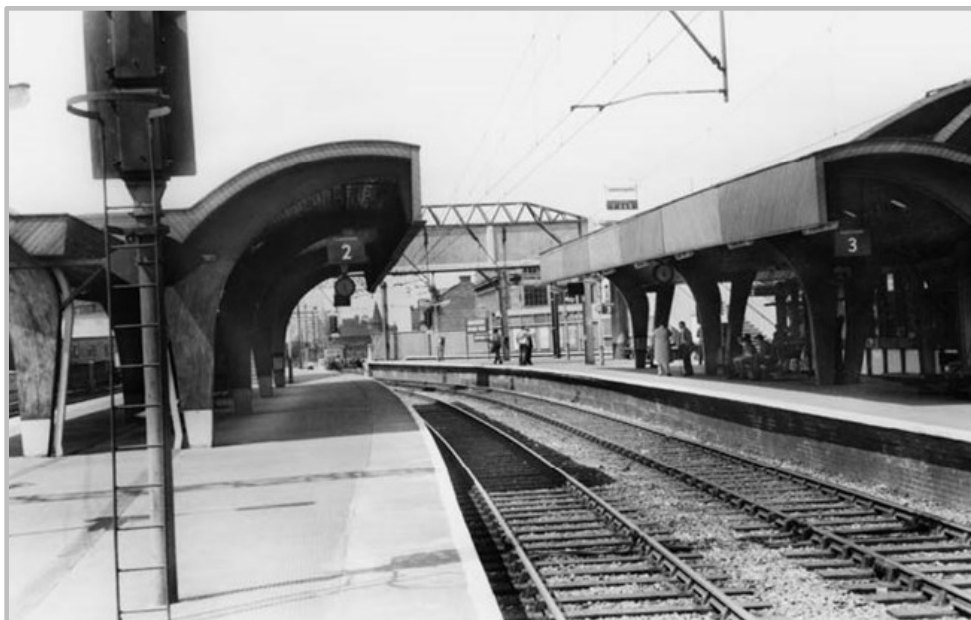
Manchester Oxford Road Platform Structures 1960's – Historic England Archive
