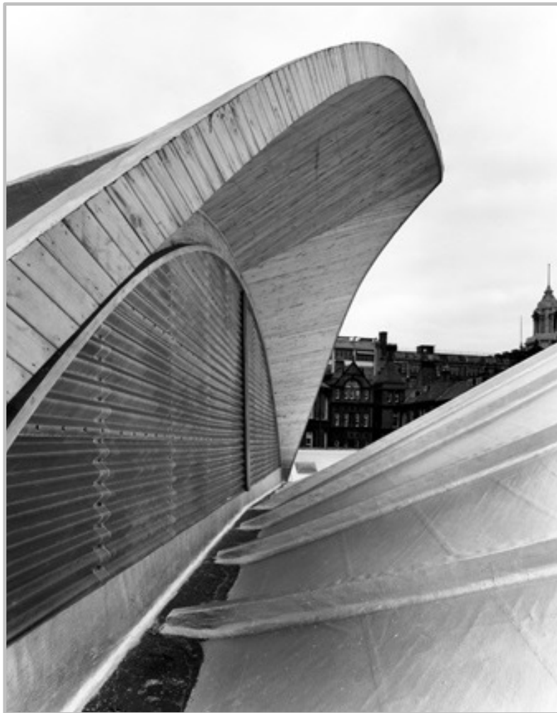
Manchester Oxford Road 1959 – Laminated Timber Shell Roof (Photo from RIBApix Ref: S59 3816)
