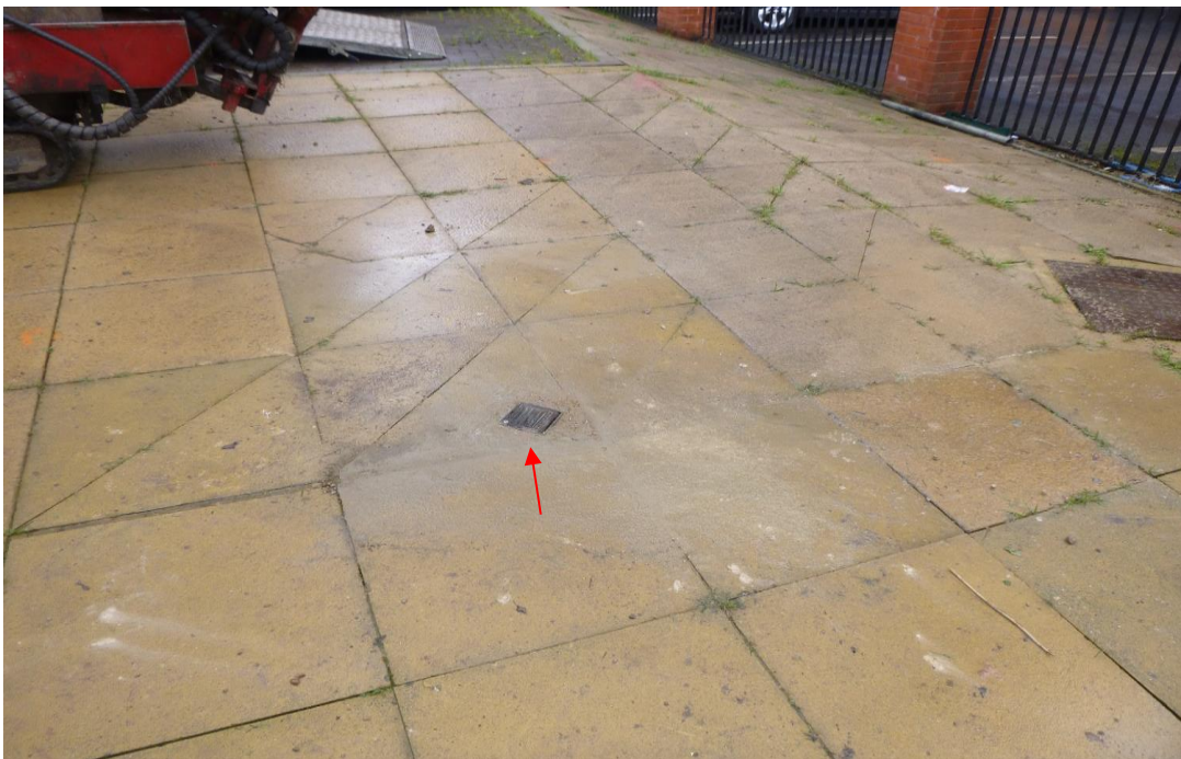
Photograph 4 Standpipe cover at the surface of WS1 after completion.
