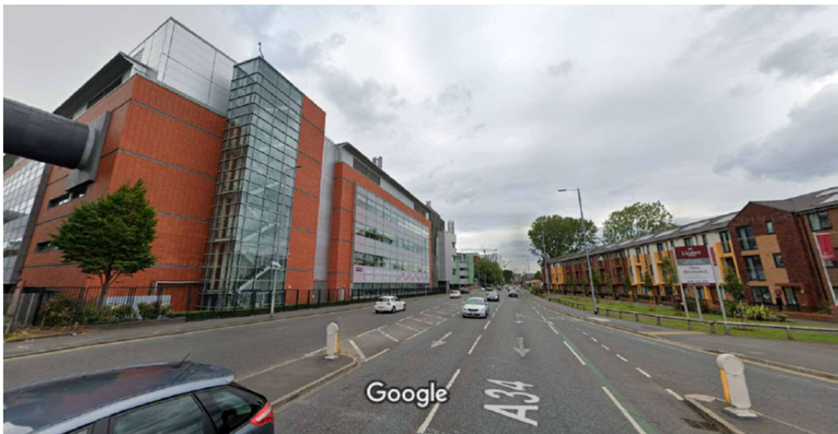
Photo 2. View of existing storage facility from Upper Brook Street
