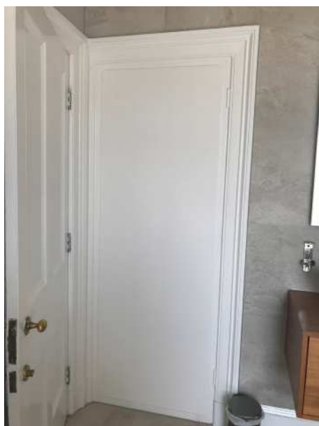
View of existing door which had been boarded
