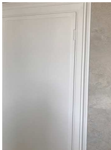
View of existing hinges to the original door
