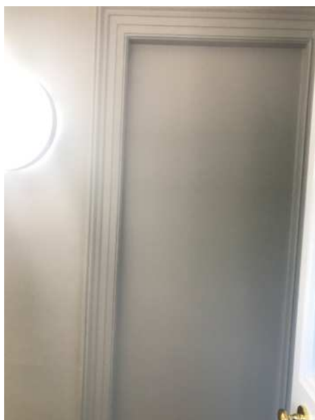
View of doorway from the staircase
