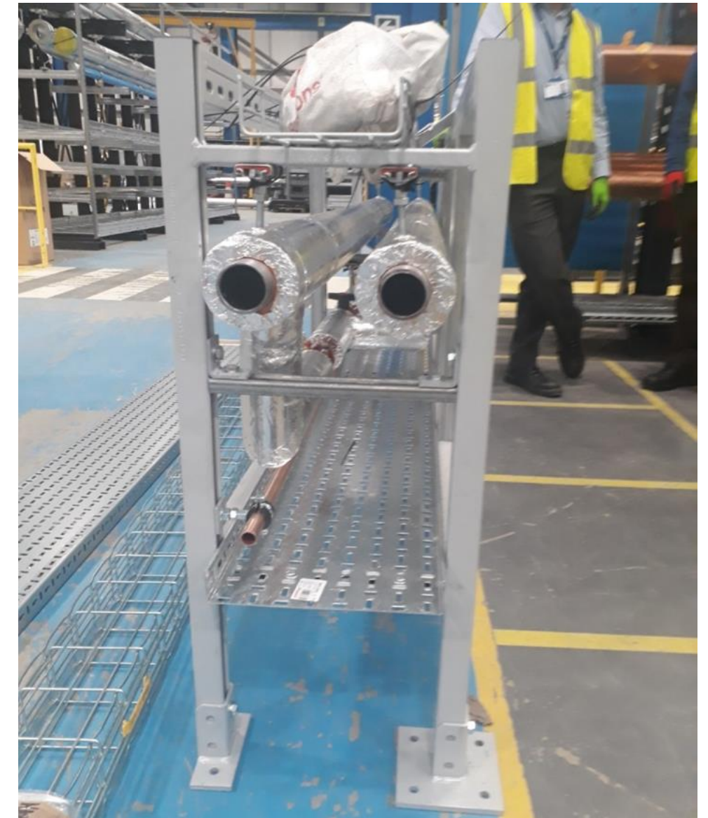
Figure 7 Example of the Unistrut as part of a mock up that was constructed
