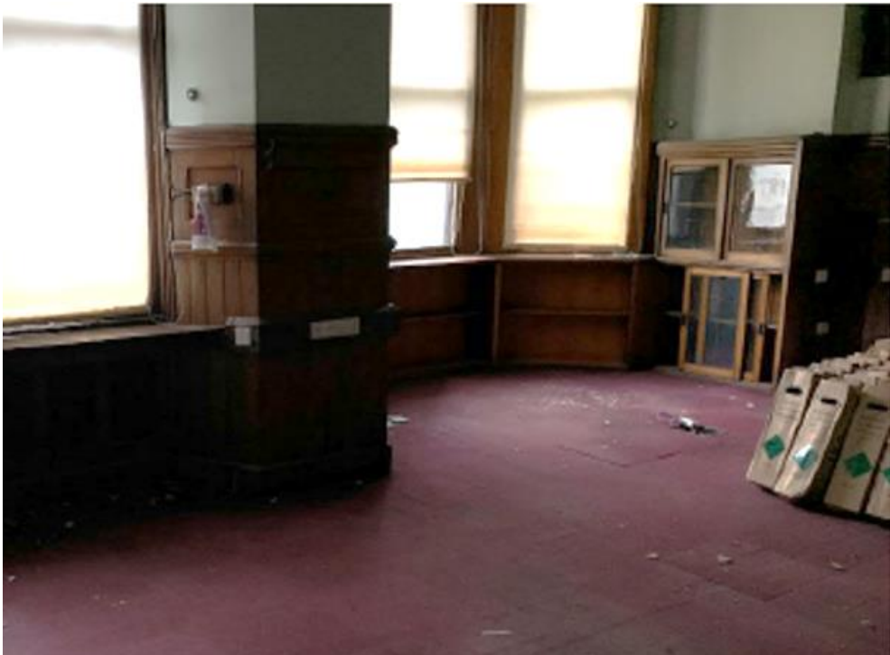
Figure 14 Example of high-quality perimeter boxing to be retained and adapted in GF-008
