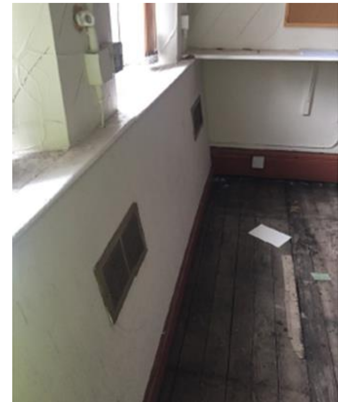
Figure 4 An example of 20th century boxing-in that would be replaced
