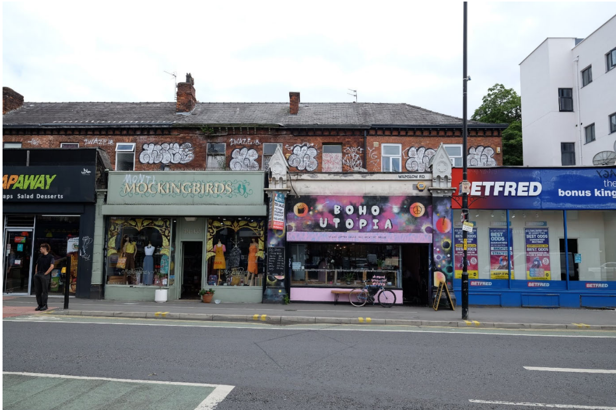
Fig 7: View across Wilmslow Road of application site.
