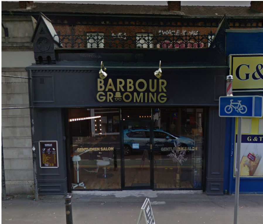
Fig 8: No. 473 Wilmslow Road (identified by BB Heritage Studio for demonstrating historic features).
