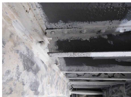
IMAGE 1 - PFC SUPPORTING DECK PLATES CORRODED AWAY MINOR CRACK IN DECK PLATE.
