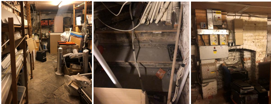
Figure 4.5: Basement to No 8 St John Street (July 2020)
