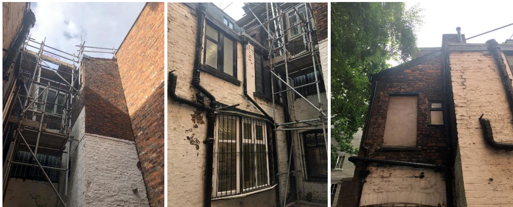
Figure 4.4: Rear Elevation to 8 and 8a St John Street (July 2020)
