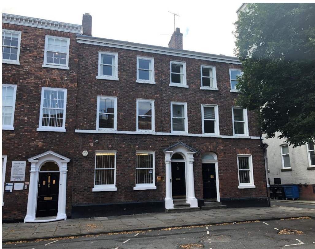
Figure 4.1: 8 and 8a St John Street (July 2020)
