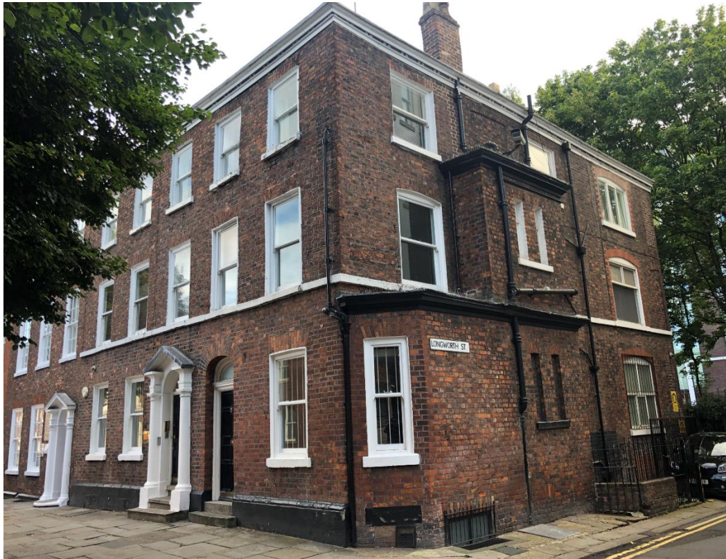
Figure 4.2: 8 and 8a St John Street (July 2020)
