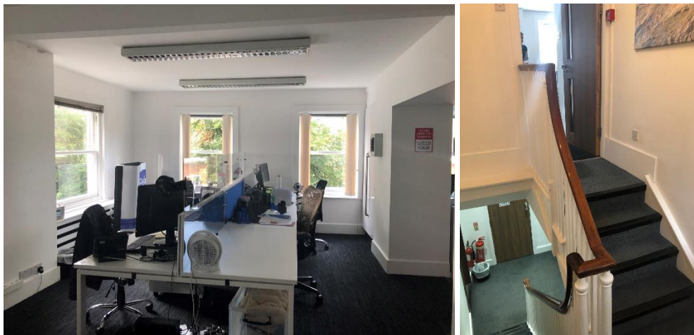
Figure 4.8: Second Floor to No 8 St John Street (July 2020)
