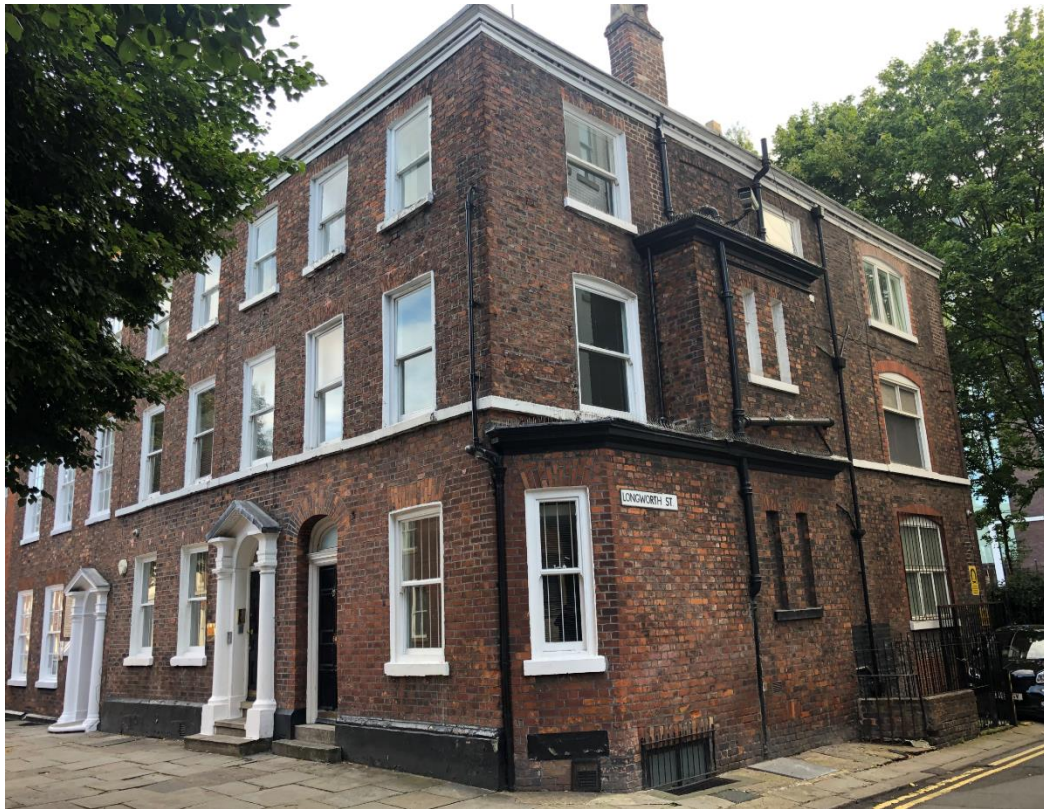
Figure 4.13: The Application Site (July 2020)
