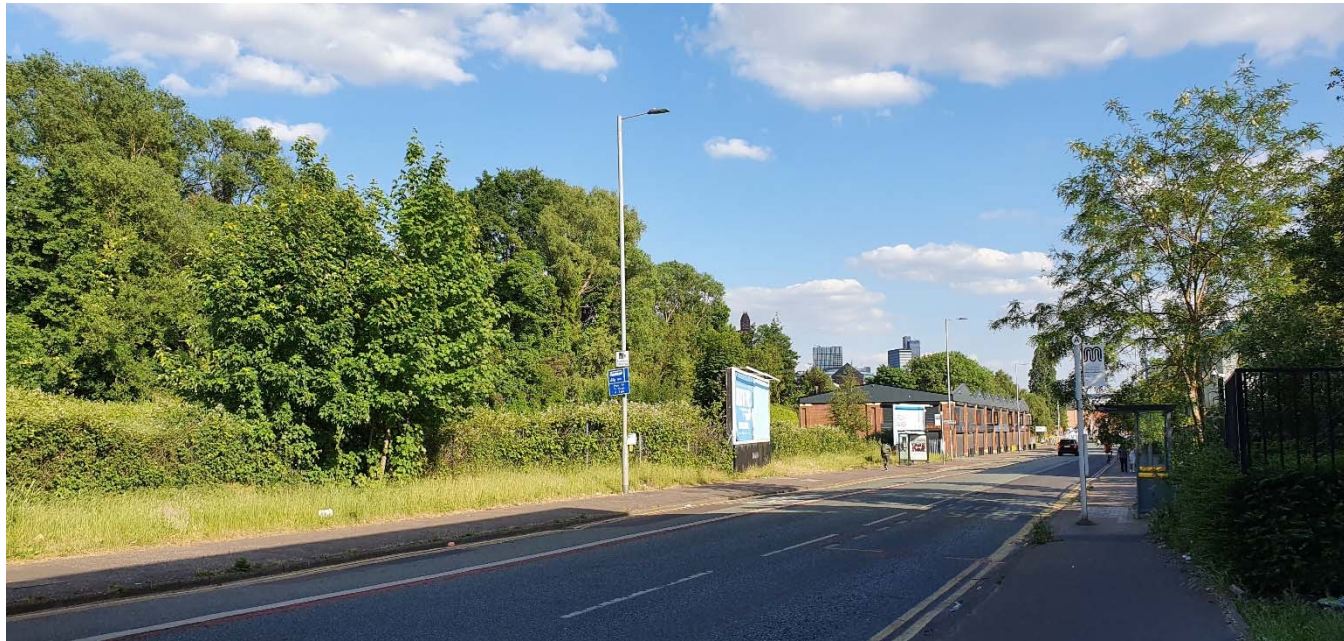
Southbound view of the development site fronting Bury New Road
