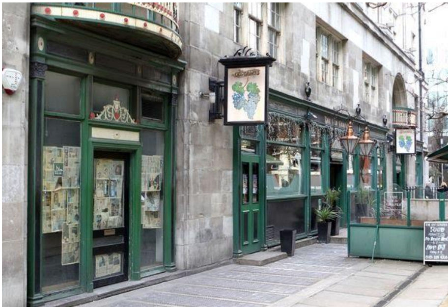
Previous Grapes Pub external elevation – which is now the new adjacent office entrance.
