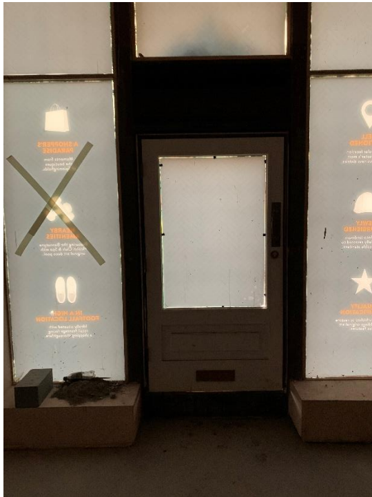
Existing doorway internal view
