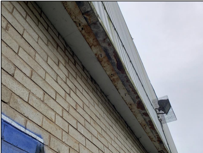
Photograph 2 showing cladding sealed to the masonry
