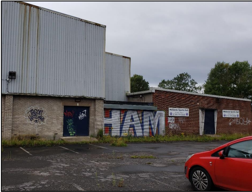
Photograph 1 showing the sports hall exterior
