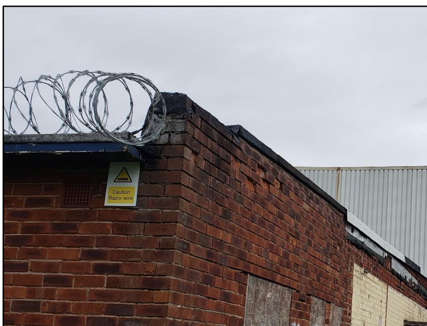
Photograph 4 showing the roof edges of the single-storey section
