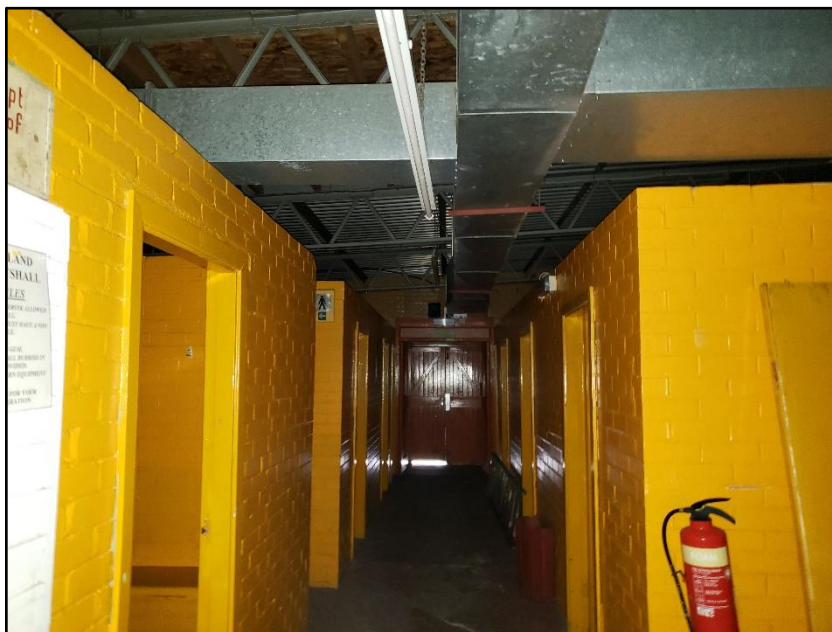
Photograph 5 showing the interior of the single-storey section
