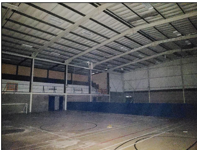
Photograph 6 showing the interior of the double-height sports hall
