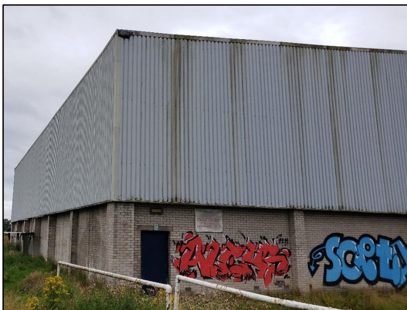
Photograph 3 showing the roof capping on the double-height section
