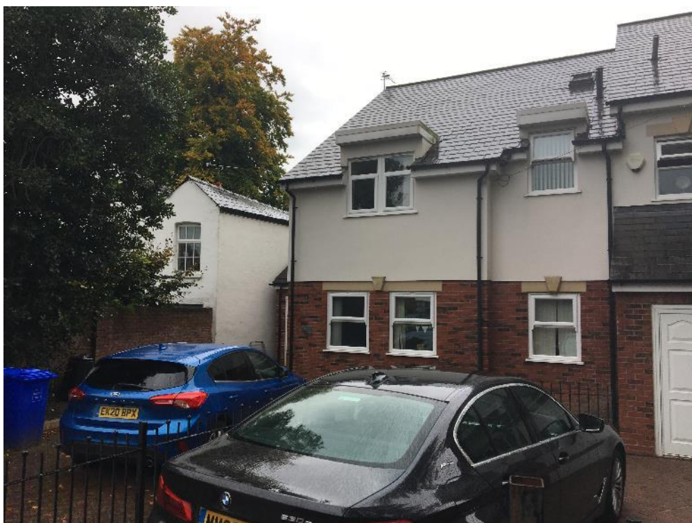
Front elevation view from right hand boundary
