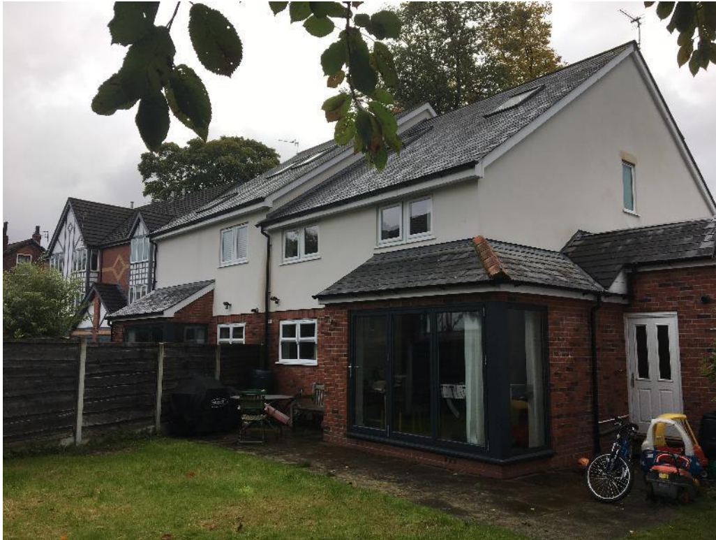
view of rear elevation and adjoining premises
