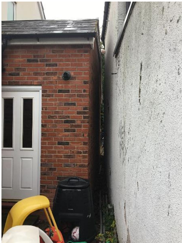
side wall of garage to boundary from rear
