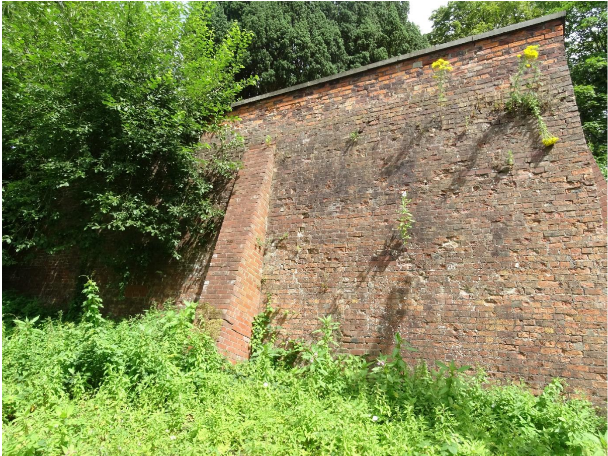
Photo 6: Retaining wall (photo taken prior to Goat Willow treatment).
