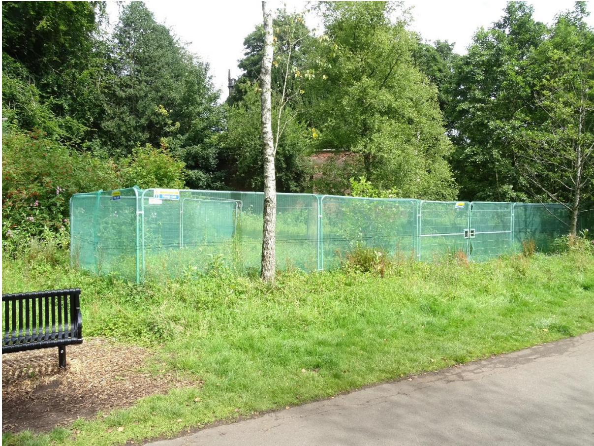
Photo 9: Temporary fencing to prevent public access to damaged wall areas
