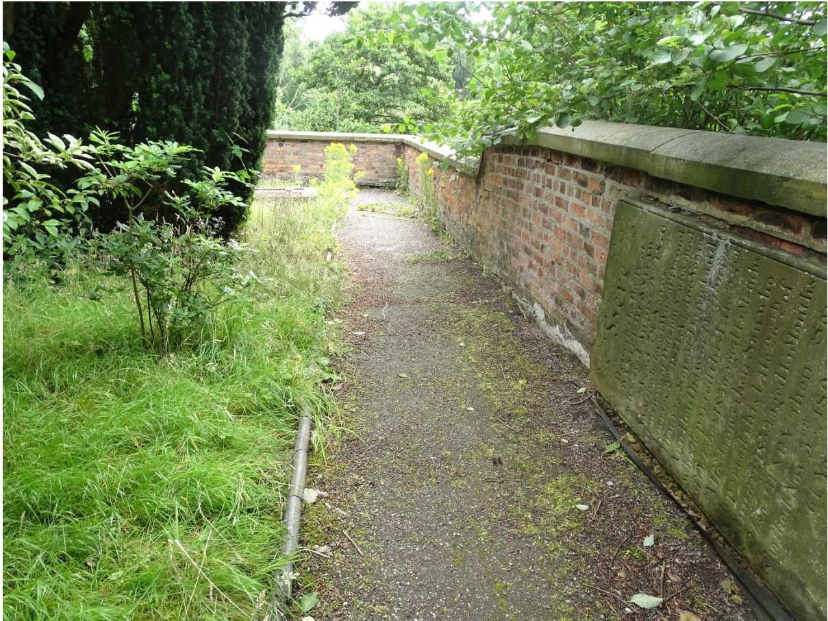
Photo 7: Existing tarmac pathway adjacent to wall.
