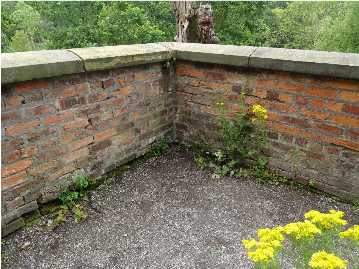
Photo 12: Section of parapet wall to be repaired and repointed
