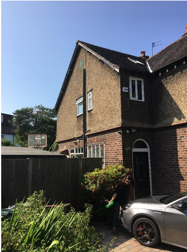
view towards side/rear from drive
