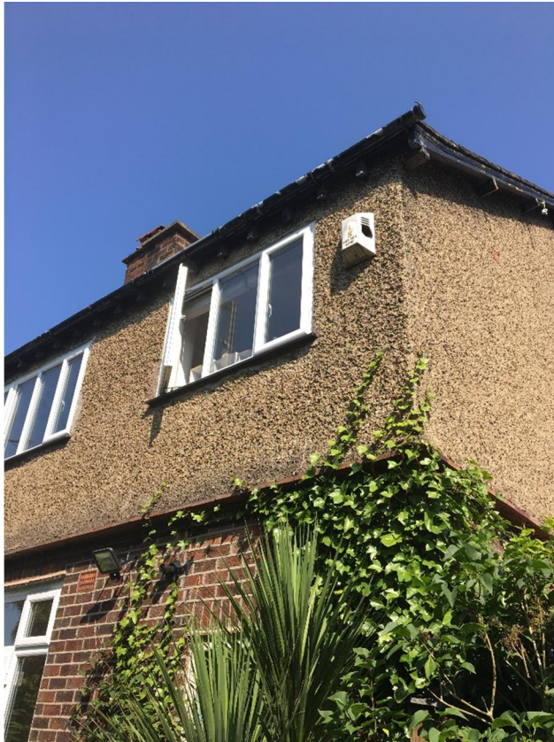
views of rear elevation
