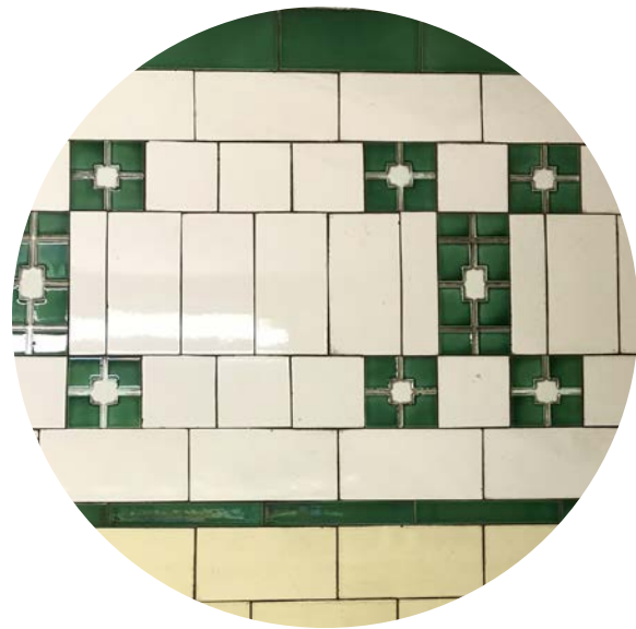
EXISTING GLAZED TILES
