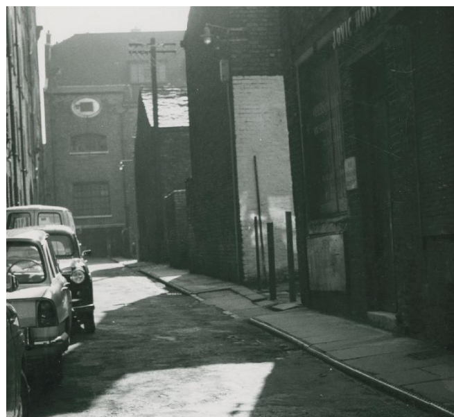
Historic view down Artillery Street looking toward the site. End of terrace visible
