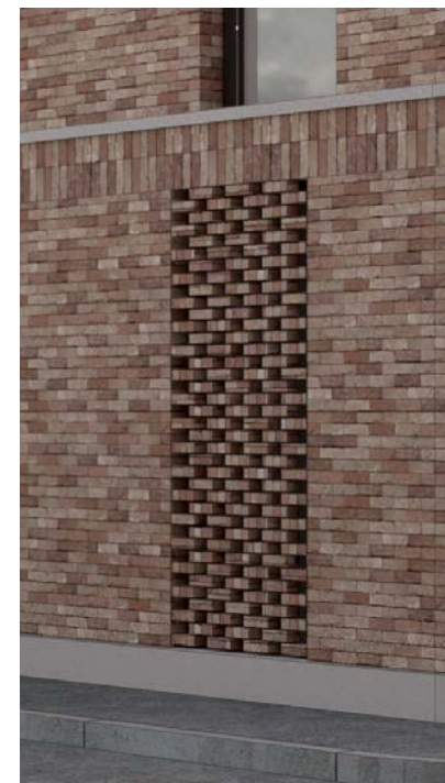
Perforated brick screening at ground level
