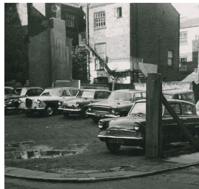
View of the rear of site from around 1965 showing the terrace houses demolished and replaced with car park
