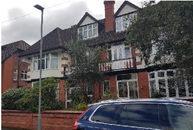
Picture of the front elevation illustrating painted ply lined dormer cheeks
