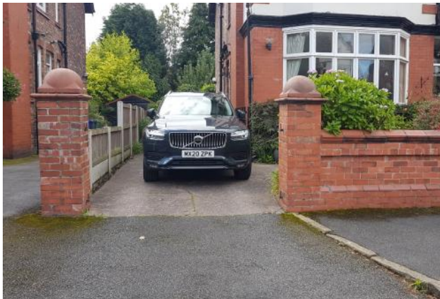
Picture of the front elevation illustrating the existing masonry piers with ornamental stone copings fronting the narrow driveway entrance.
