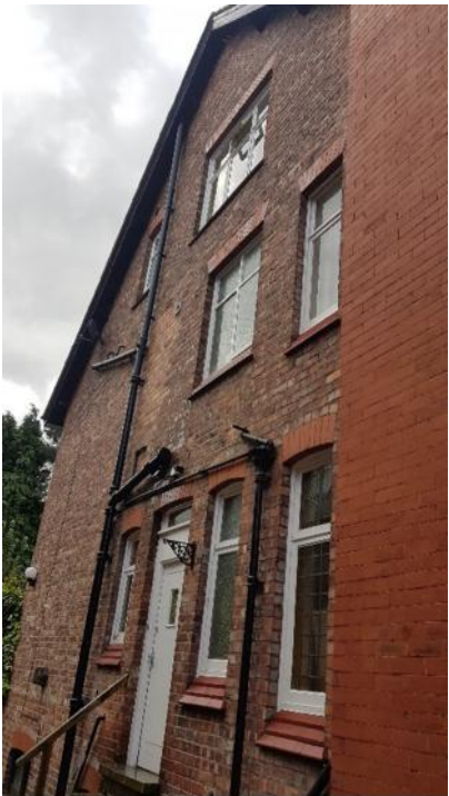
Picture of the side elevation illustrating the kitchen door and side window
