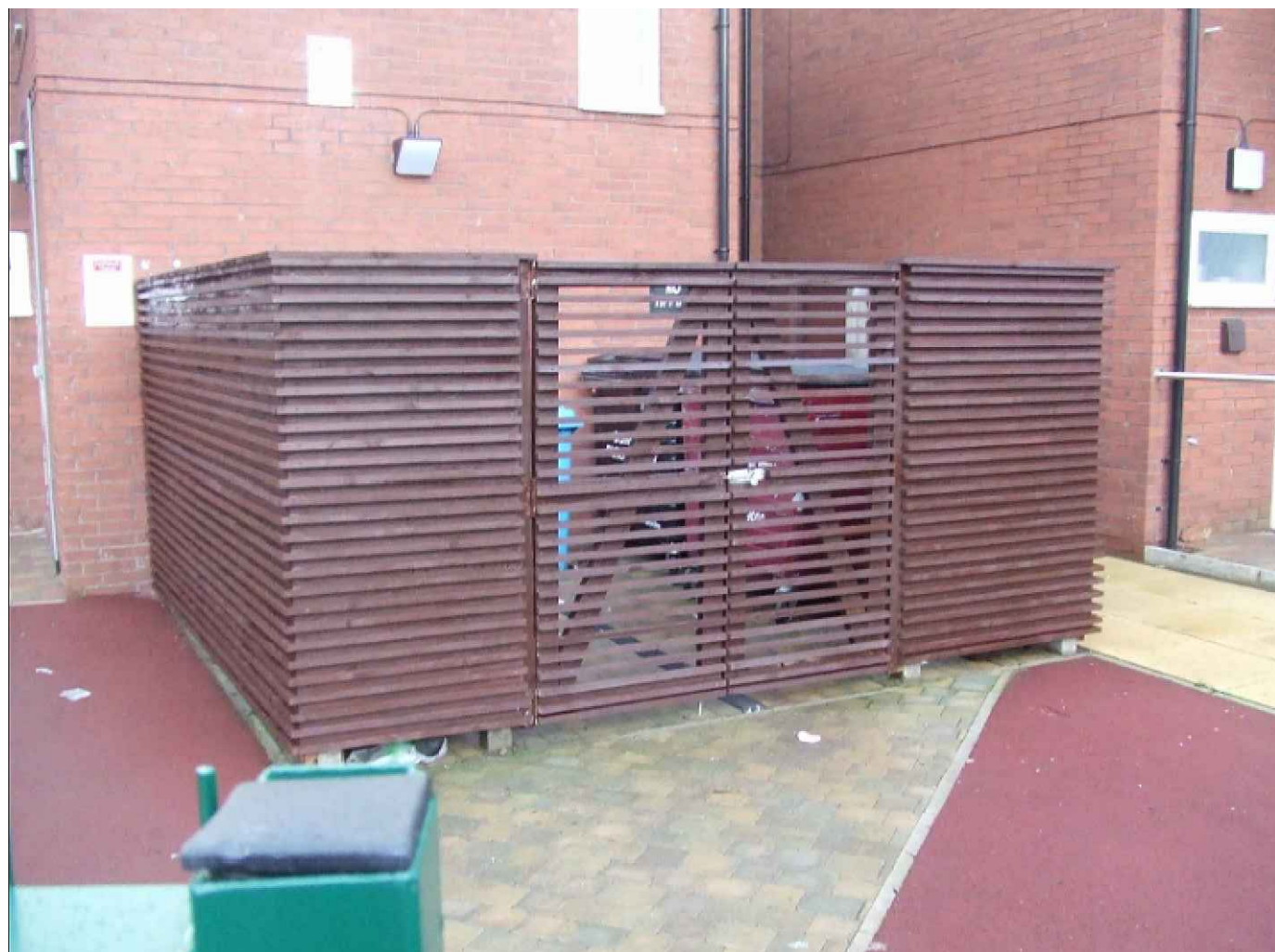
New Bin Storage
