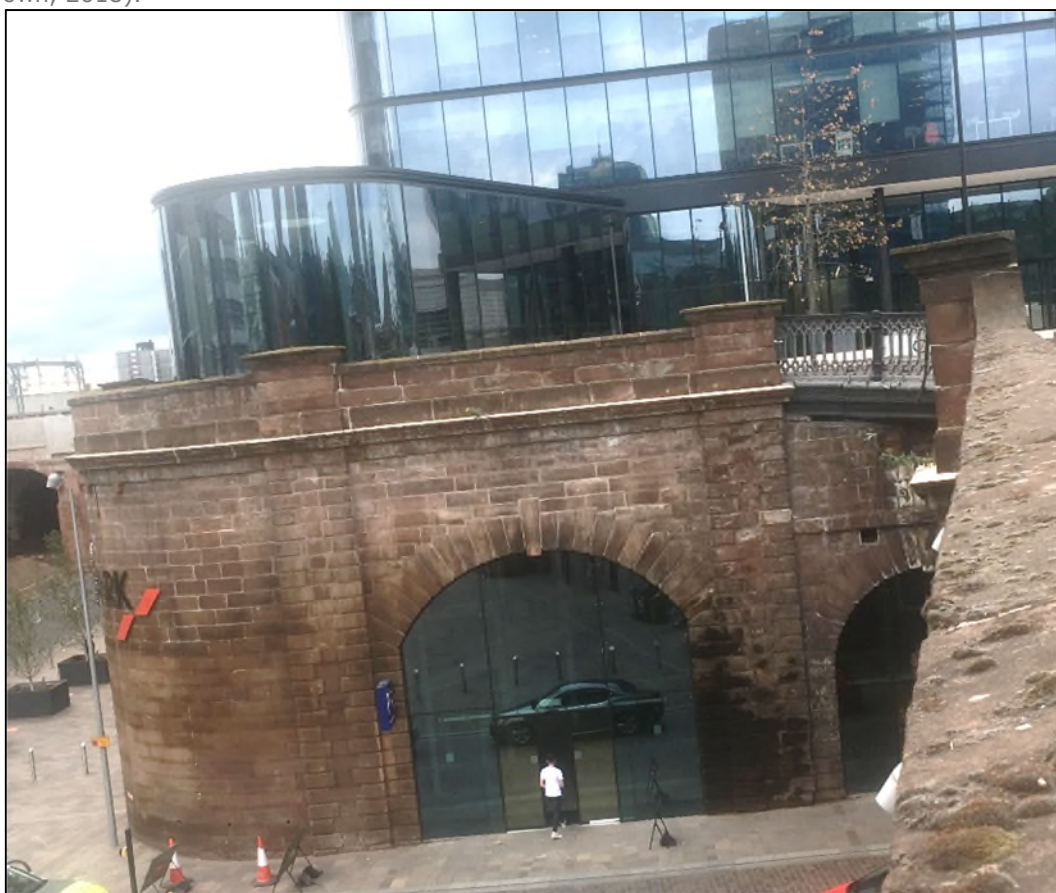
Figure 4.12: View from the Cathedral Approach bridge looking northwest towards the Railway Viaduct. (Author's own, 2018).
