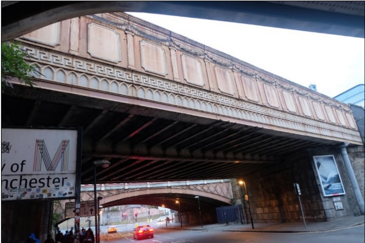
Figure 4.17: View from Victoria Street/ Great Ducie Street (A56) looking south towards the Middle Bridge. (Author's own, 2018).
