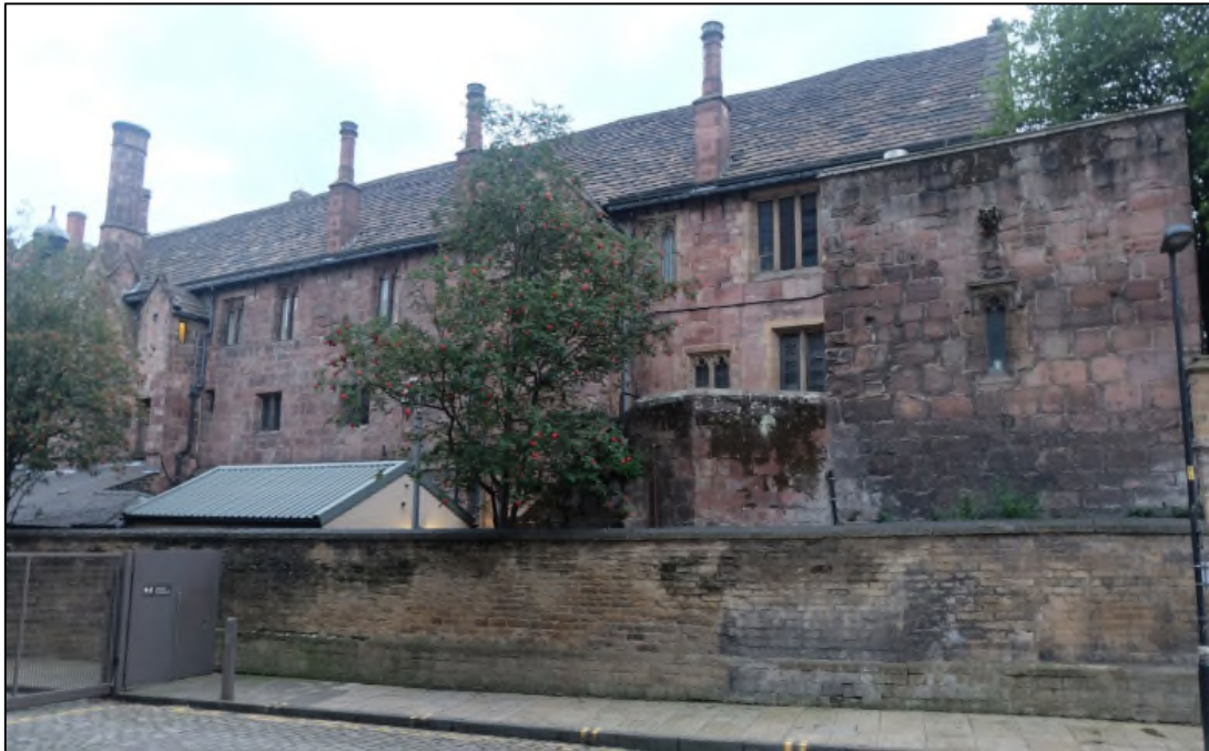
Figure 4.3: Top photograph taken from Hunts Bank / Walker's Croft junction looking south towards the Chetham's Hospital and attached wall. Bottom photograph taken from inside the Chetham's complex looking north towards the Chetham's Library and hospital building. (Author's own, 2018).
