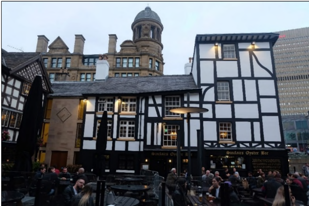
Figure 4.10: (Left) View from Exchange Square/ New Cathedral Street looking north towards Sinclairs Oyster Bar. (Author’s own, 2018).
