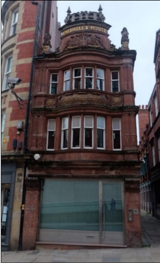
Figure 4.7: View on Cateaton Street looking north towards Mynshulls House. (Author's own, 2018).
