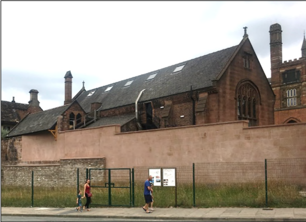
Figure 4.4: Top photograph - view from Victoria Street looking east towards the detached block of the schoolroom. Bottom photograph – view looking north at the school room building from inside the Chetham's complex. (Author's own, 2018).
