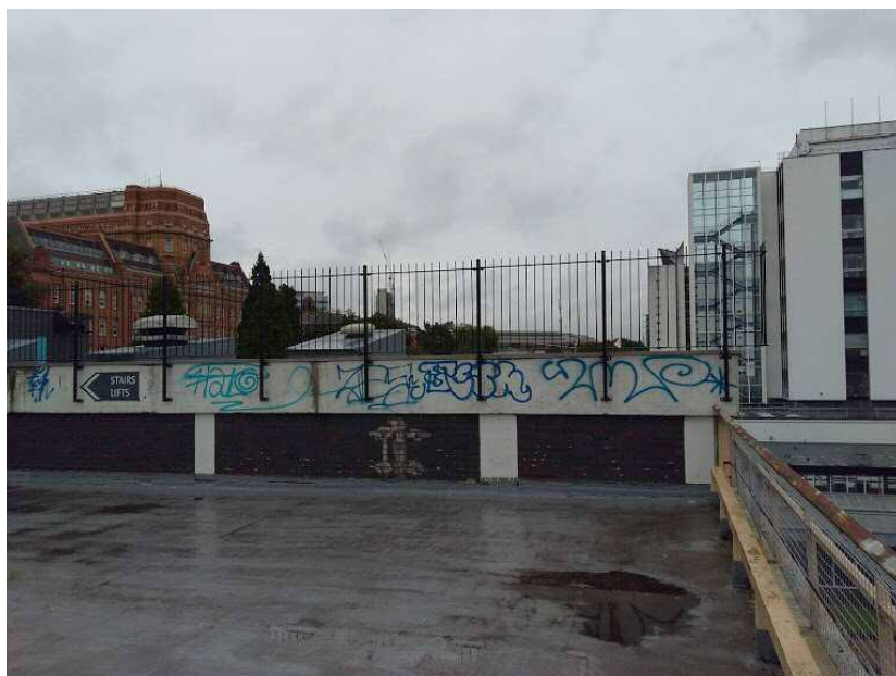
Photo 15. Existing rooftop fencing
