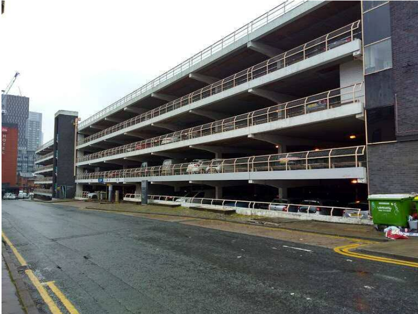
Photo 3. Existing South elevation on Charles Street
