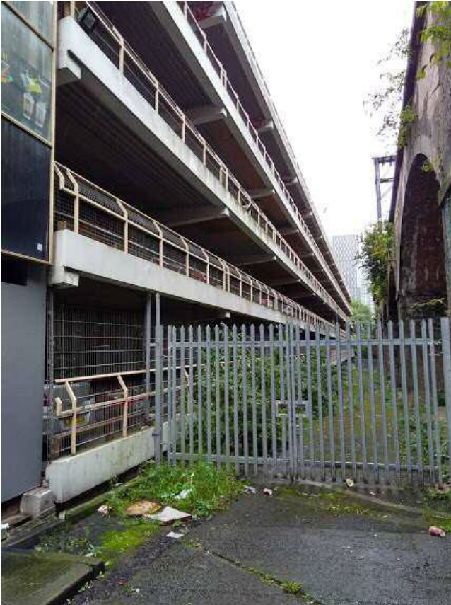
Photo 1. Existing North elevations off Sackville Street
