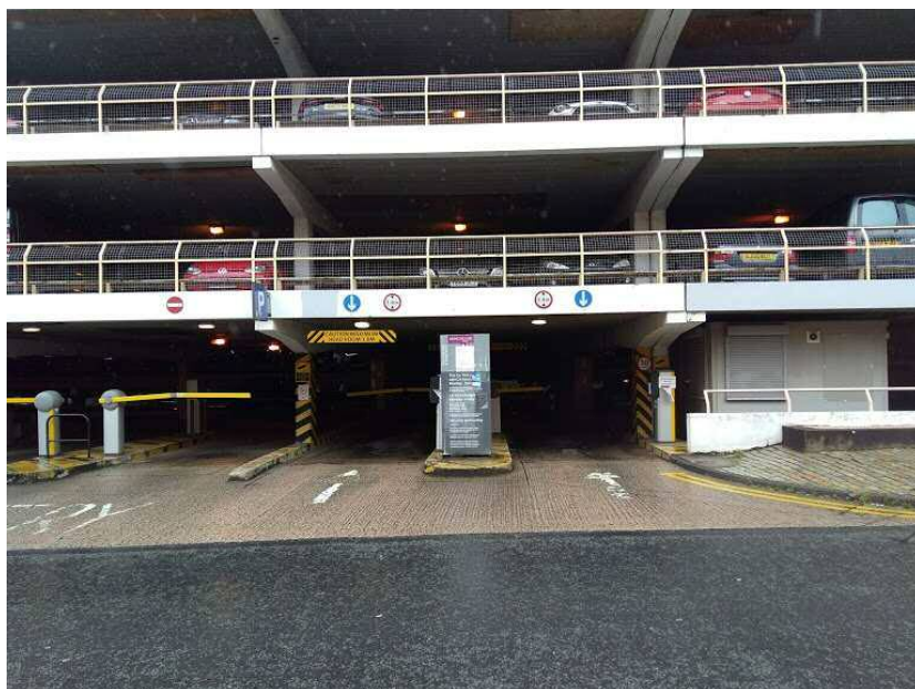
Photo 9. Existing entrance off Charles Street
