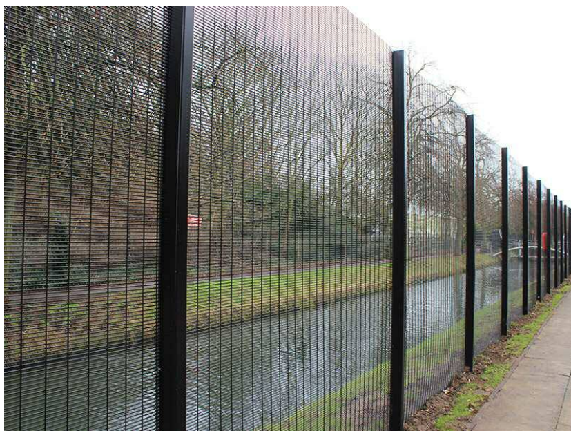
Photo 17. Example of type of anti-climb weld mesh fencing proposed
