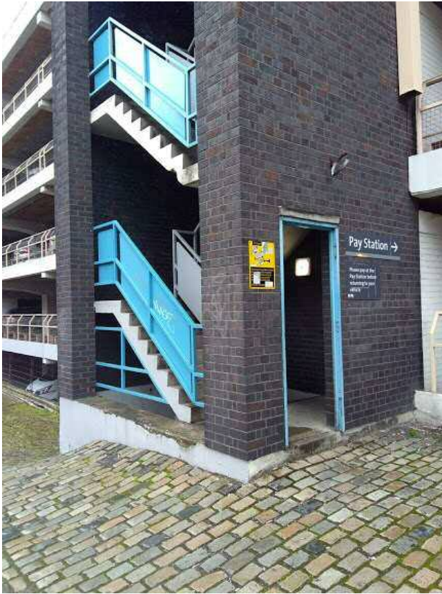
Photo 11. Existing stairs on Charles Street
