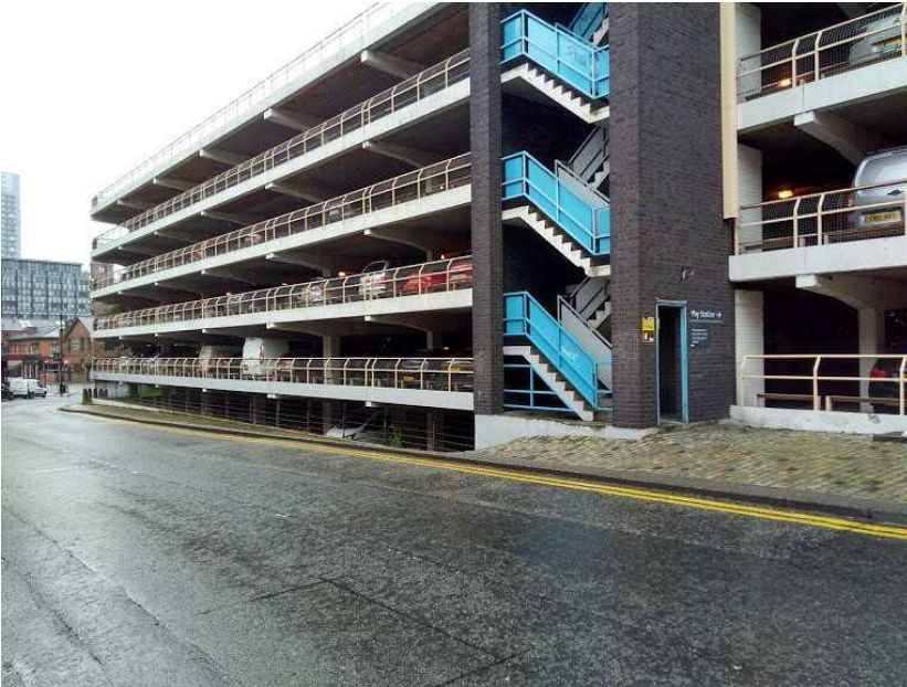
Photo 4. Bottom half of existing South elevation on Charles Street
