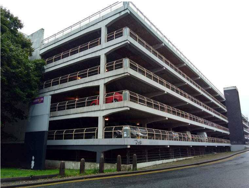
Photo 5. Existing South West corner on Charles Street
