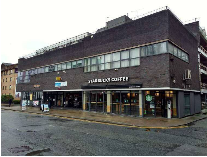
Photo 2. Existing East elevation on Sackville Street
