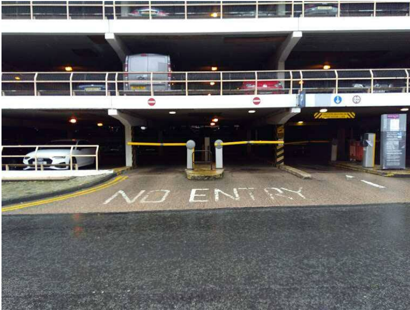
Photo 10. Existing exit off Charles Street
