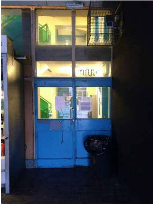
Photo 12. Existing pedestrian entrance off Sackville Street
