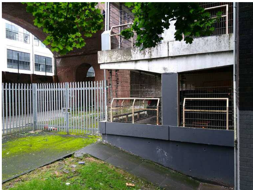
Photo 8. Existing West elevation to left of staircase
