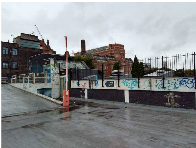
Photo 14. Existing rooftop fencing
