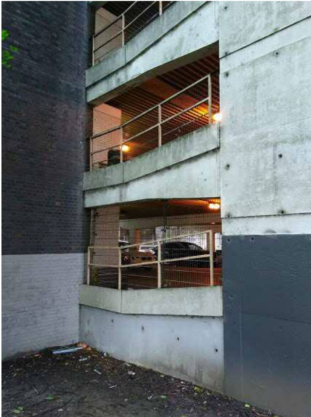
Photo 6. Existing West elevation to right of staircase
