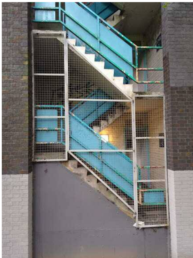
Photo 7. Existing West elevation staircase
