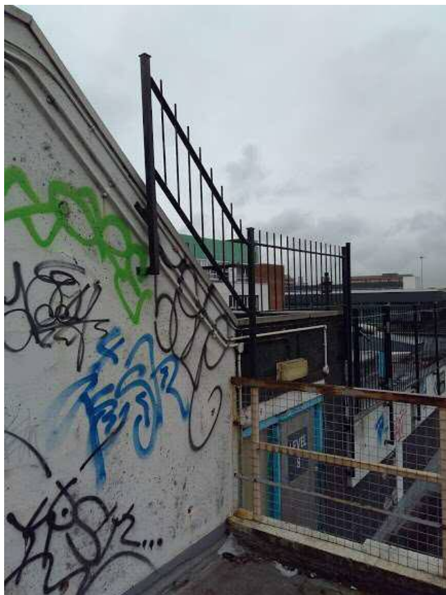
Photo 13. Existing rooftop fencing
