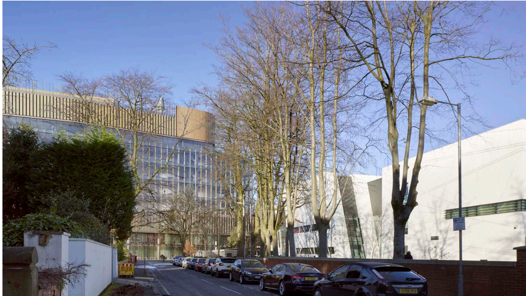
Representative View 13 View from Kinnaird Road towards the East Elevation Planning Approved
