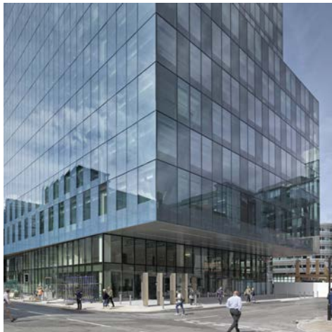
No 1 Spinningfields, Manchester, Simpson Hough Architects
