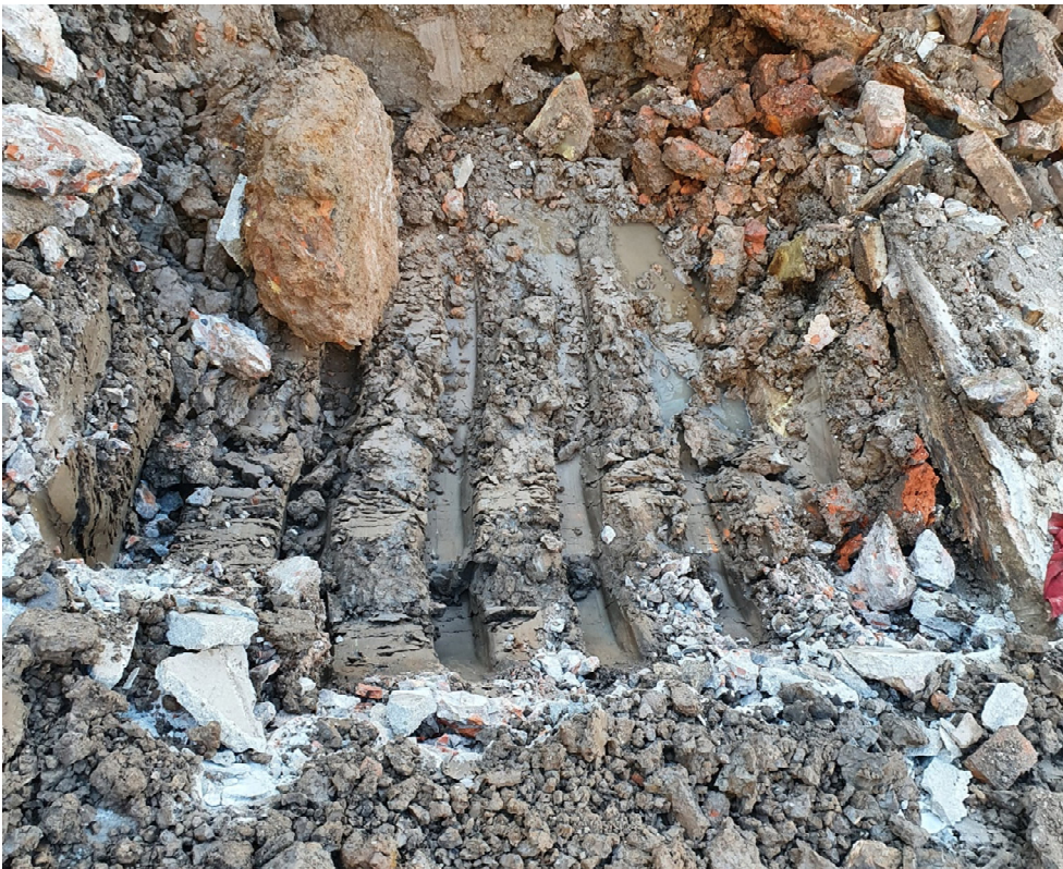
Photograph 3 – Natural soils exposed beneath basement in TP101
