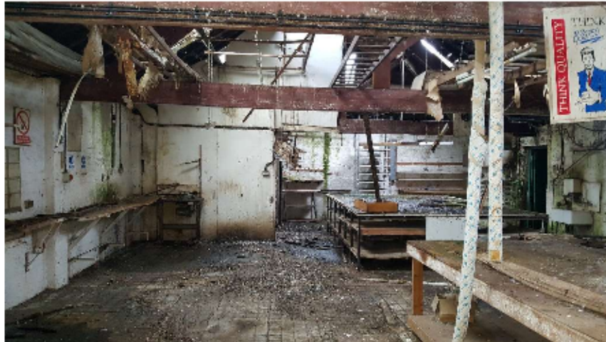
King post trusses
