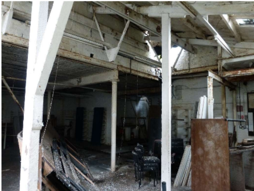
Concrete mezzanine floor supported on steel beams and circular posts together with the timber roof and supporting posts to the lean-to building.
