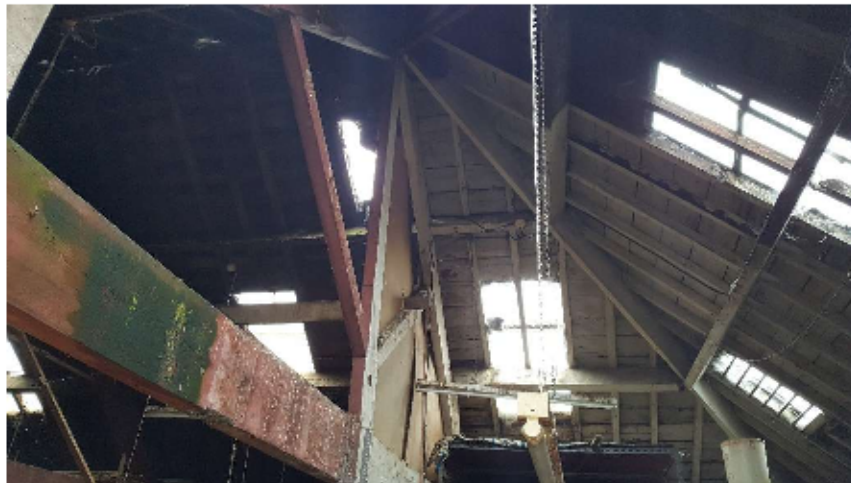
Timber hip members with timber boards to the roof
