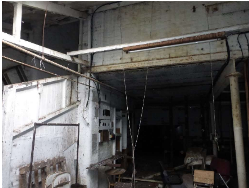
Production building first floor beams and columns. Note access ramp to left
