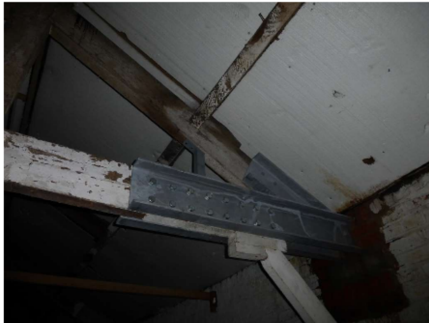
Covered access – repairs to all timber truss ends
