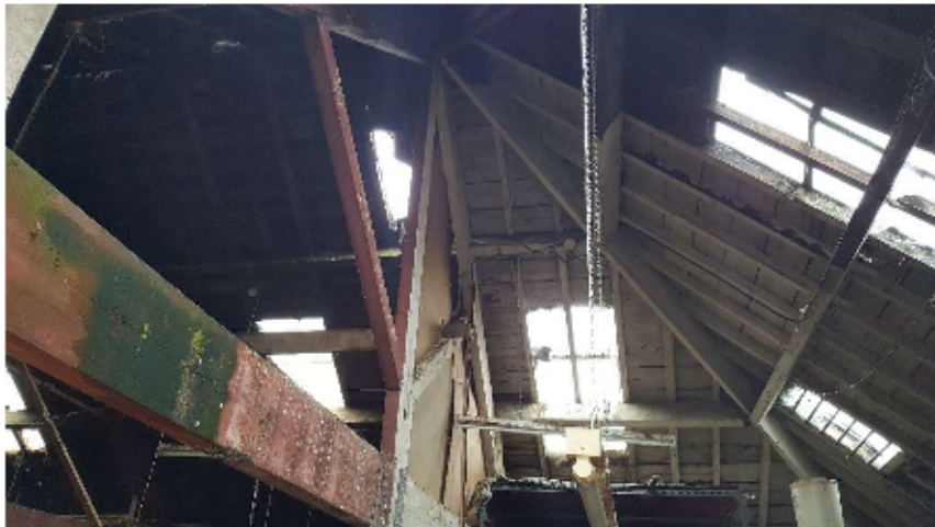
Hipped construction at both ends in 2017
