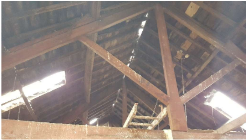
Detailed view of the roof construction in 2017
