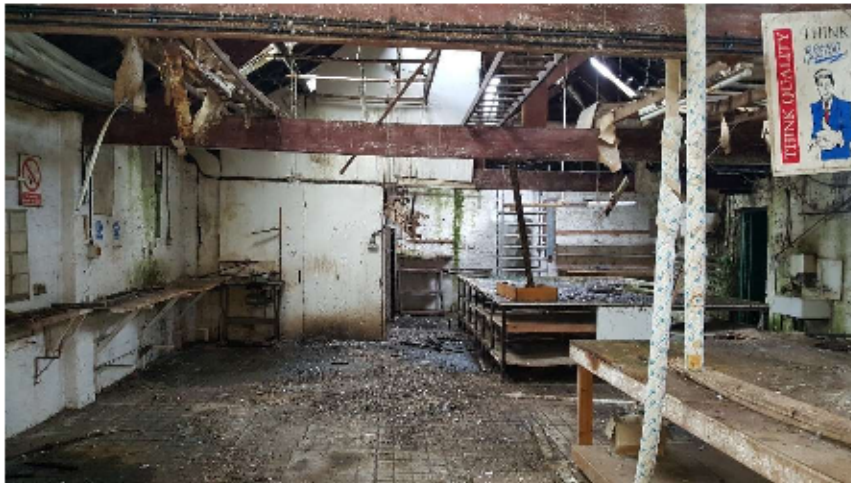
Mezzanine floor with timber truss roof above in 2016
