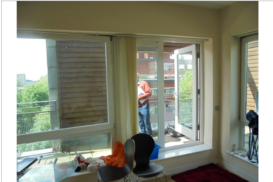
Photograph: 05 Description: Internal timber framed windows in Apartment 23 overlooking Oxford Road.
