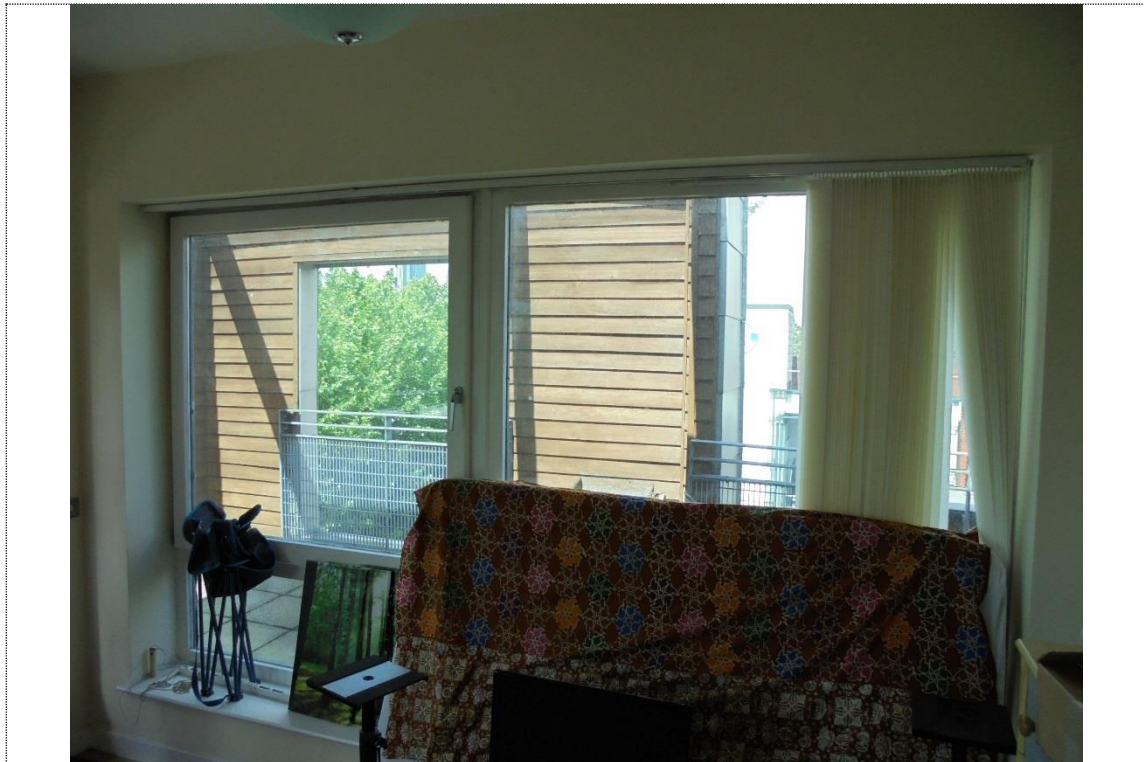
Photograph: 06 Description: Internal timber framed windows in Apartment 23 overlooking Sydney Street.
