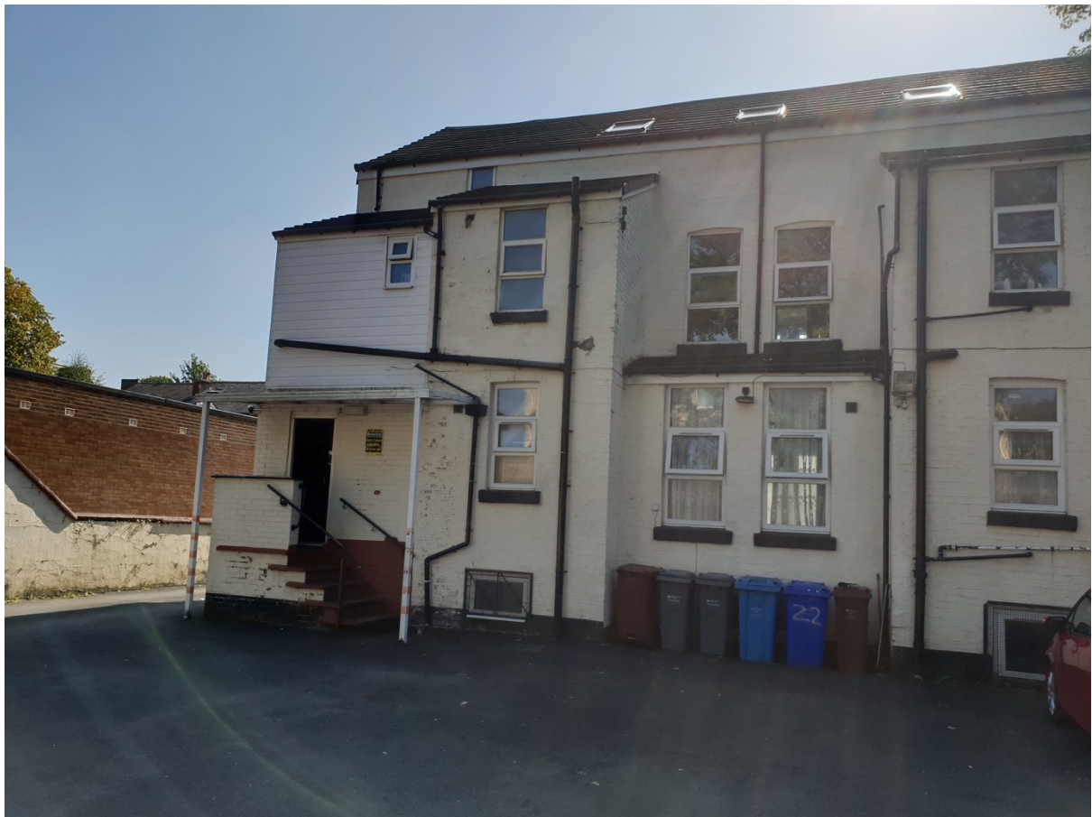
Image 2: Existing view of rear elevation from Car Park.
