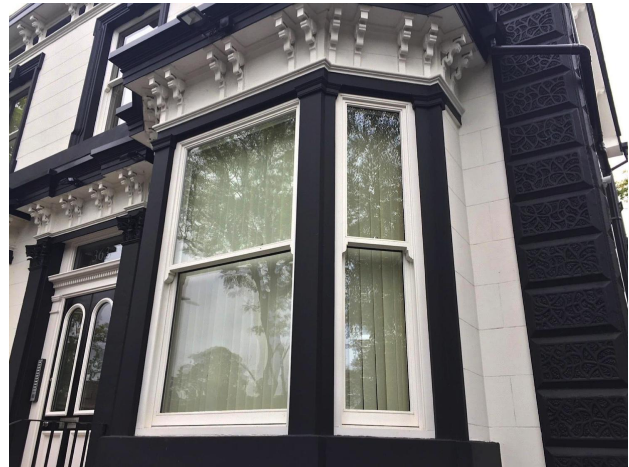
Replacement windows as completed in 2016
