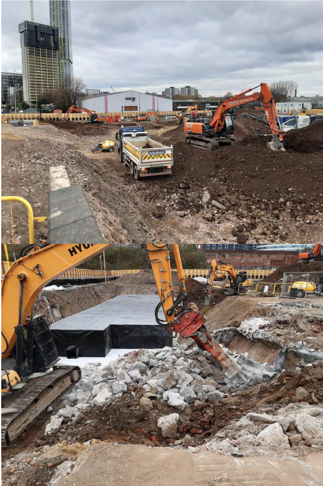
Removal of material from Area 5. Removal of USTs in Area 2.
