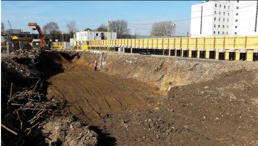
Area 1B ready for attenuation tank. Oversize stockpile in Area 1C for crushing into southern boundary
