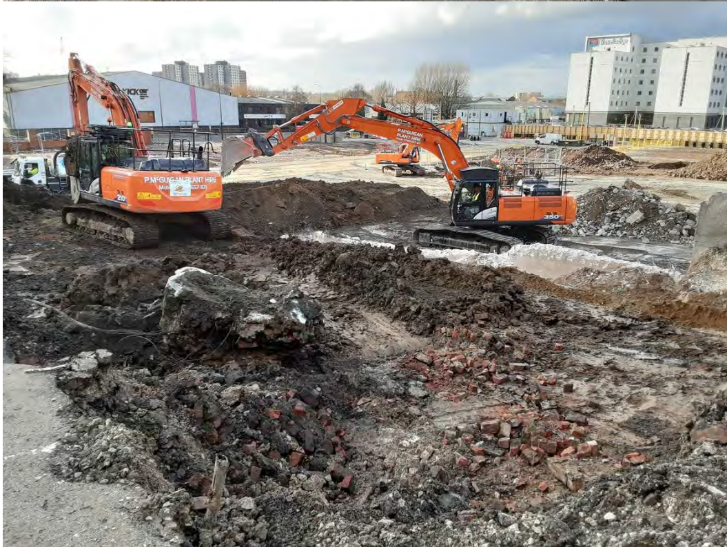
Demolition of retaining wall in Area 1A with oversize and made ground stockpiled in Area 7 to be crushed.
