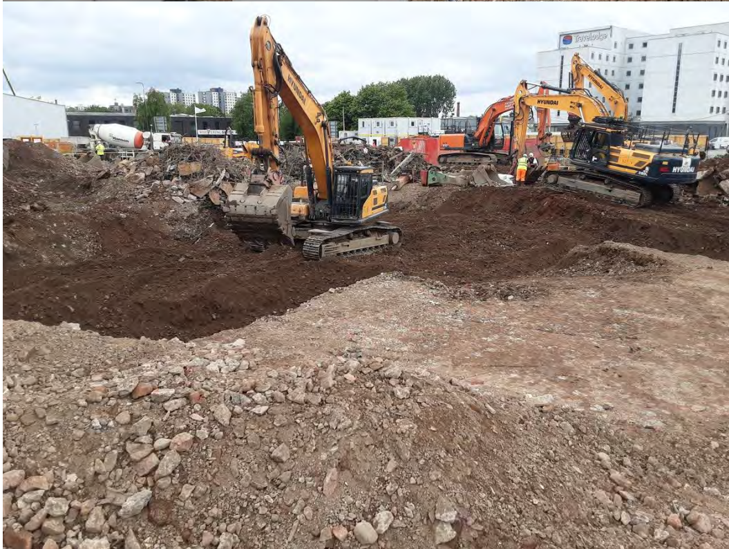
Construction of ramp. Placement of material in Areas 4 & 5.
