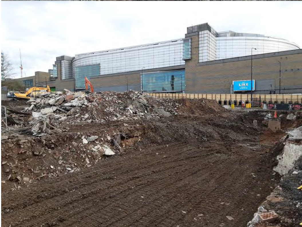
Area 1B & Area 1C. Stockpiling of oversize in Area 3A for processing.
