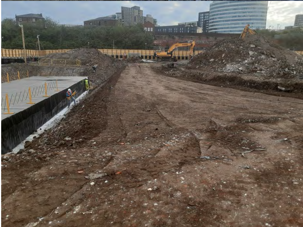
Crushing from oversize in Area 4 into Area 7. Placement of material in Area 3B
