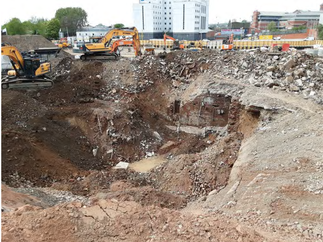
Crusher in Area 6 discharging to Area 7. Former abstraction well located in Area 6.
