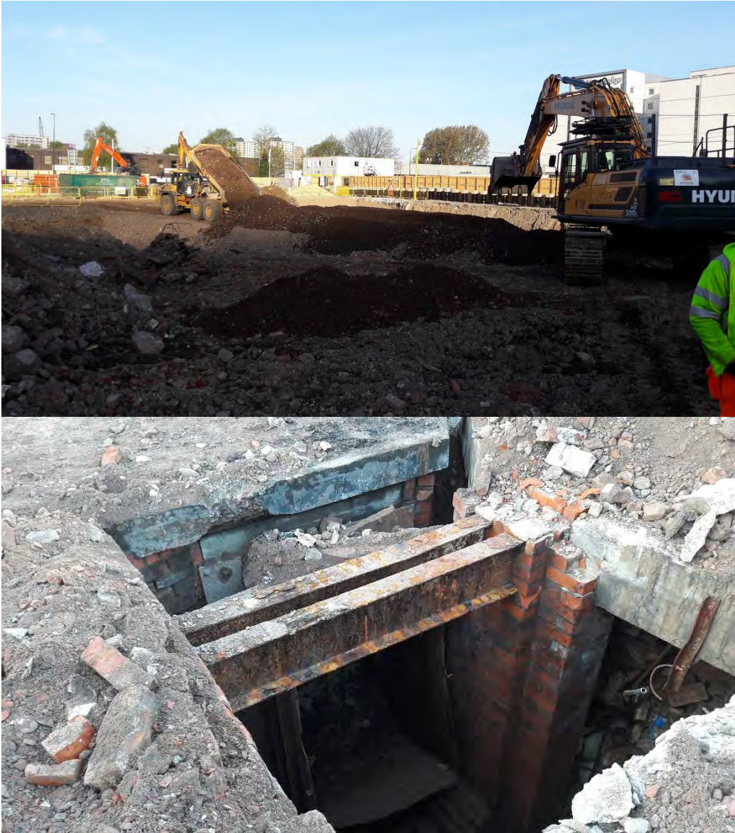
Continued placement in Area 3B. Discovery of significant voids in Area 6.
