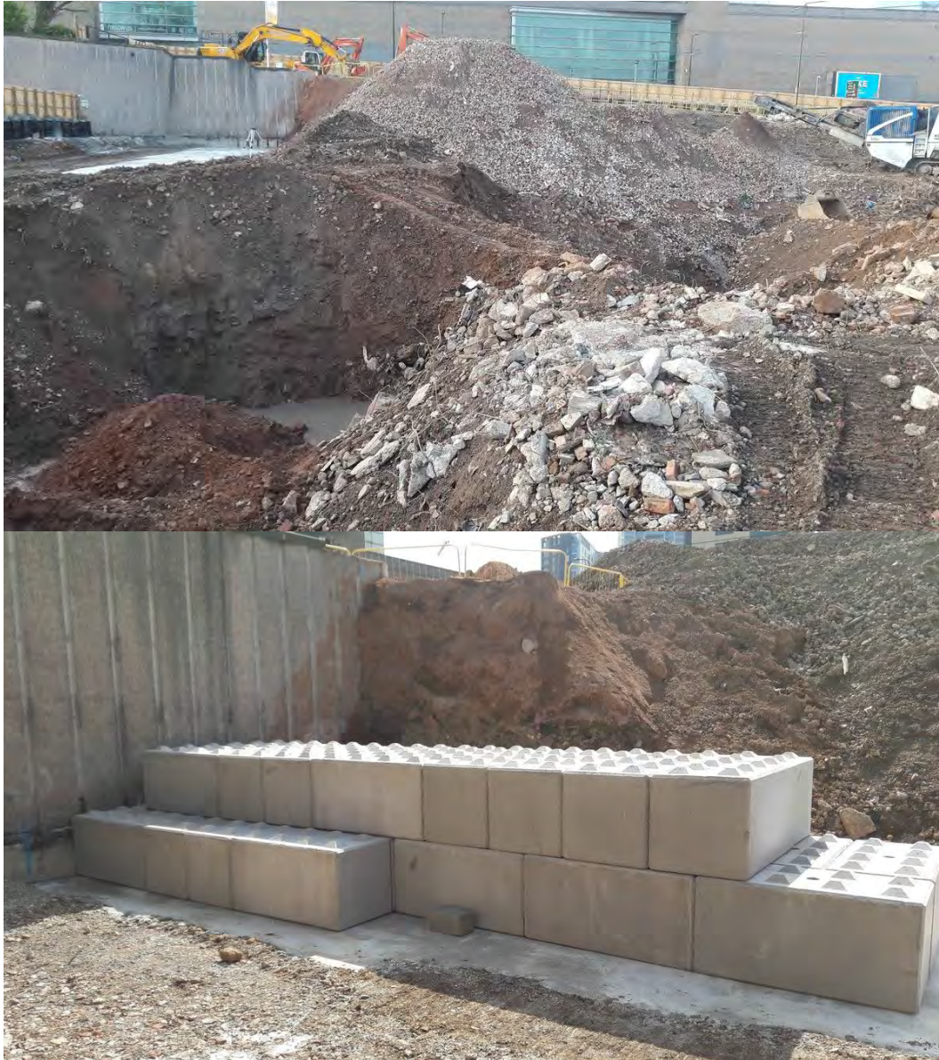
Excavation of green strip and placement of block wall.
