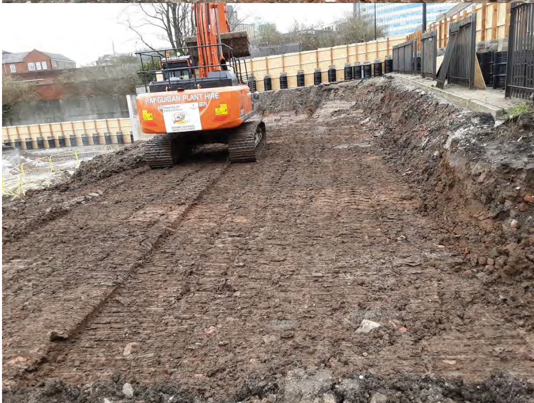
Formation of ramp in Area 1A. Excavate Area 6.
