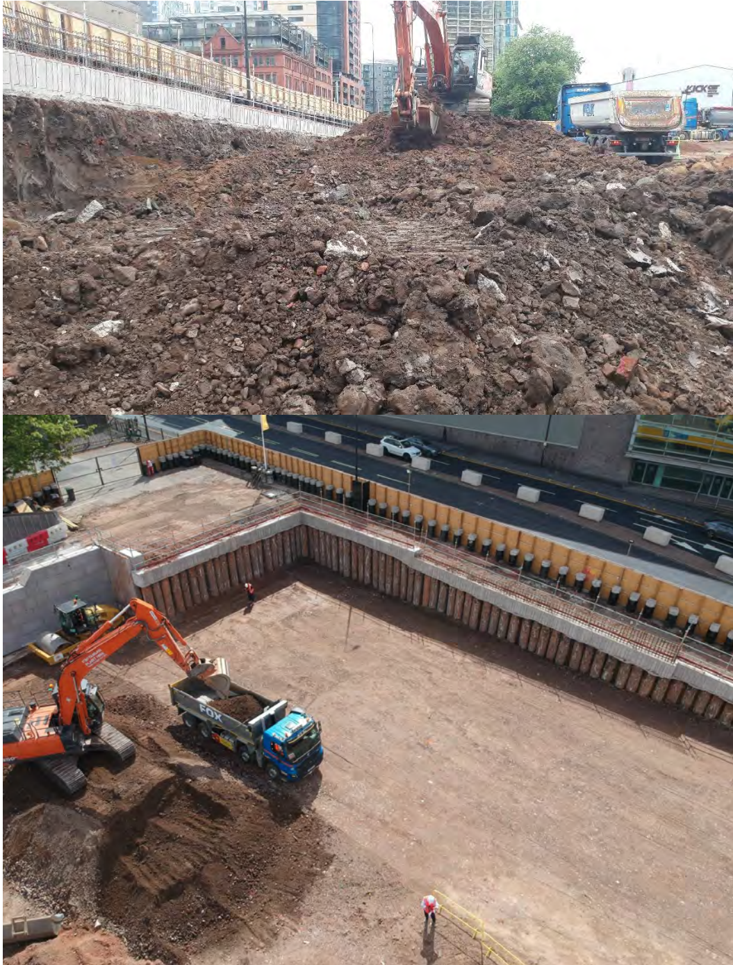
Removal of temporary piling ramp (Area 1A) to form site levels (Area 8). Surplus removed by Fox Brothers Ltd.
