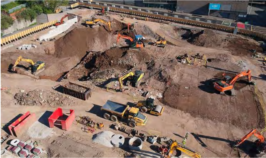
Aerial view showing excavation of made ground, stockpiles of different materials, sorting and formation of site levels.
