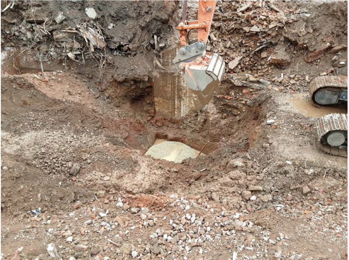
Bentonite pellets installed into abstraction well.
