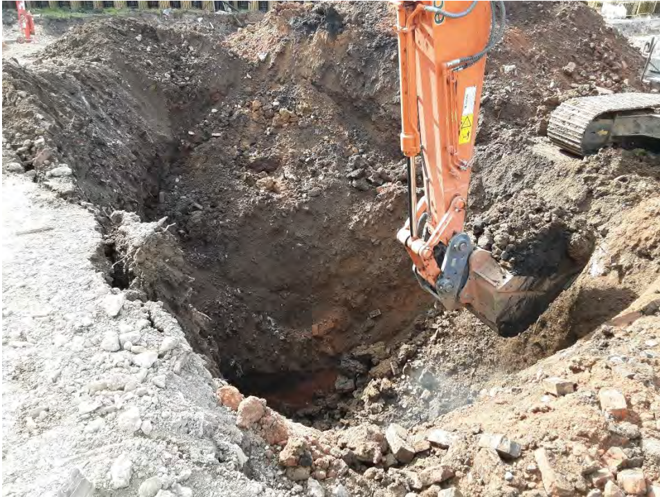
Example of grubbing out of relict in-ground structures in made ground.
