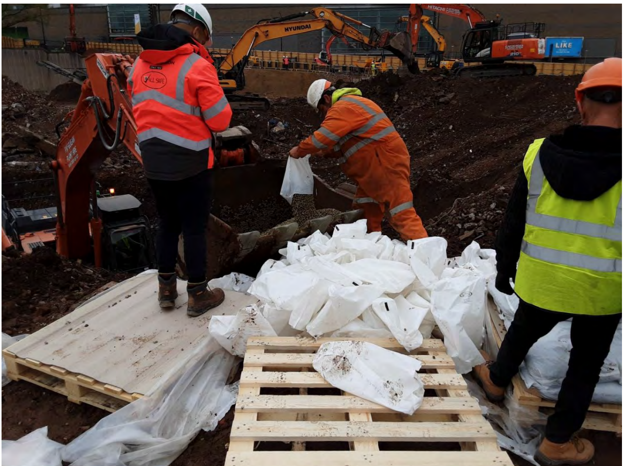
4m 3 of bentonite pellets being loaded into excavator bucket.
