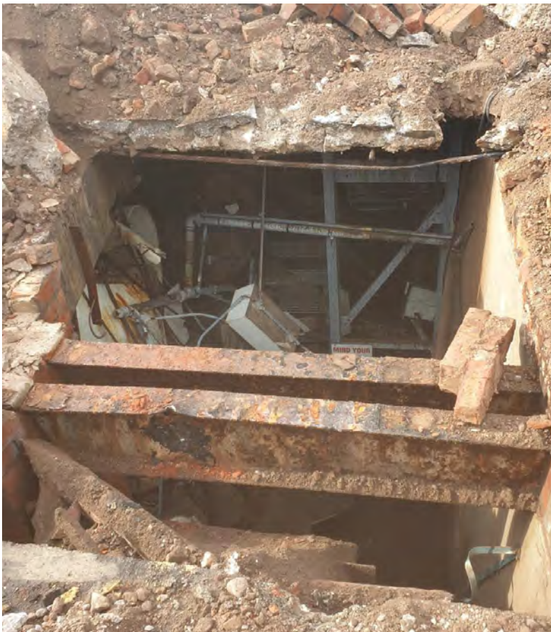
Example of subterranean basement voids and relict structures encountered during enabling works.
