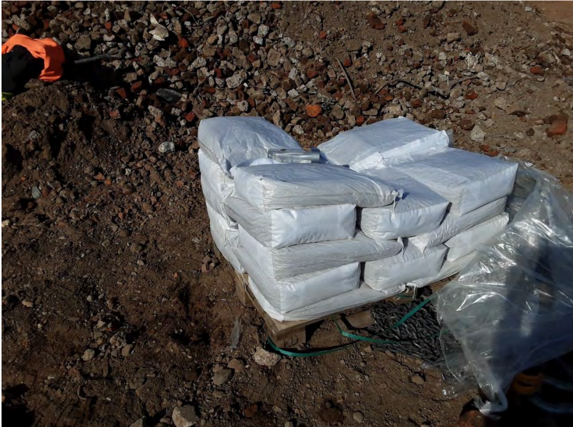
Bentonite ready to be installed into abstraction well.
