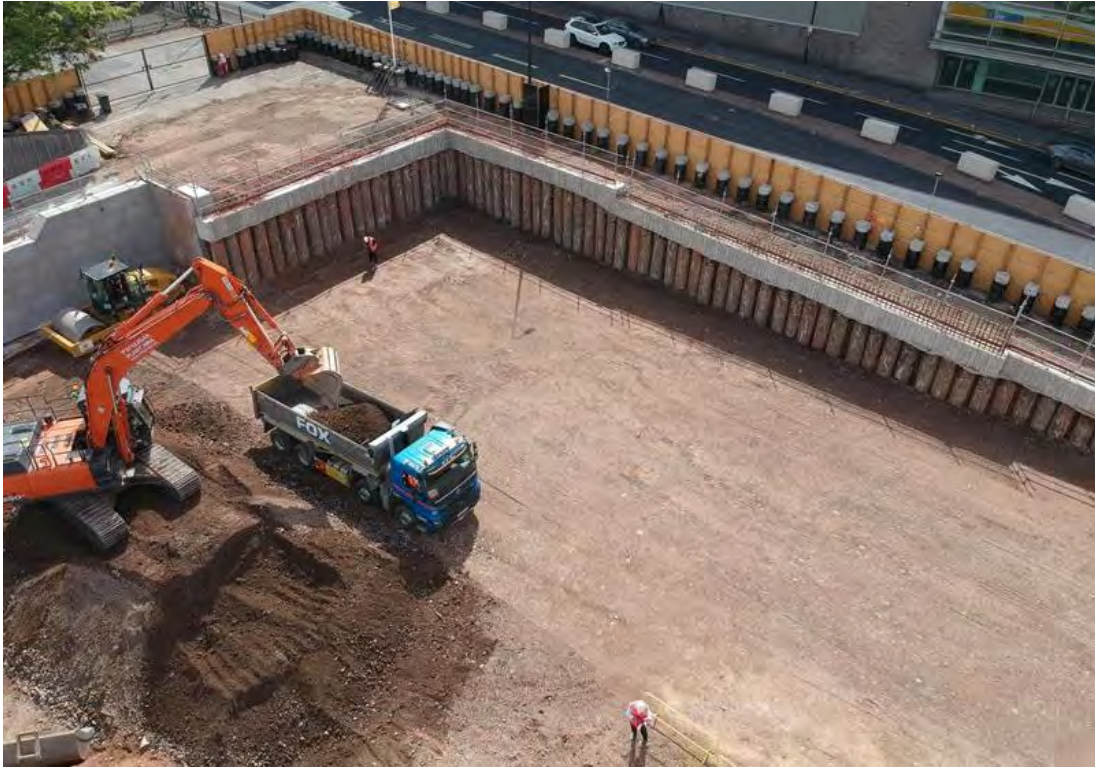
Aerial view showing surplus soils removed from site and remediated site levels.
