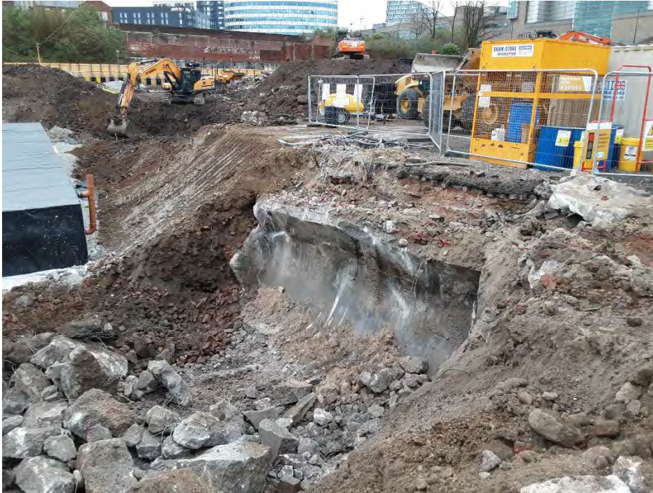
Remnants of concrete surrounds visible following removal of UST. No evidence of spillage/leakage identified.
