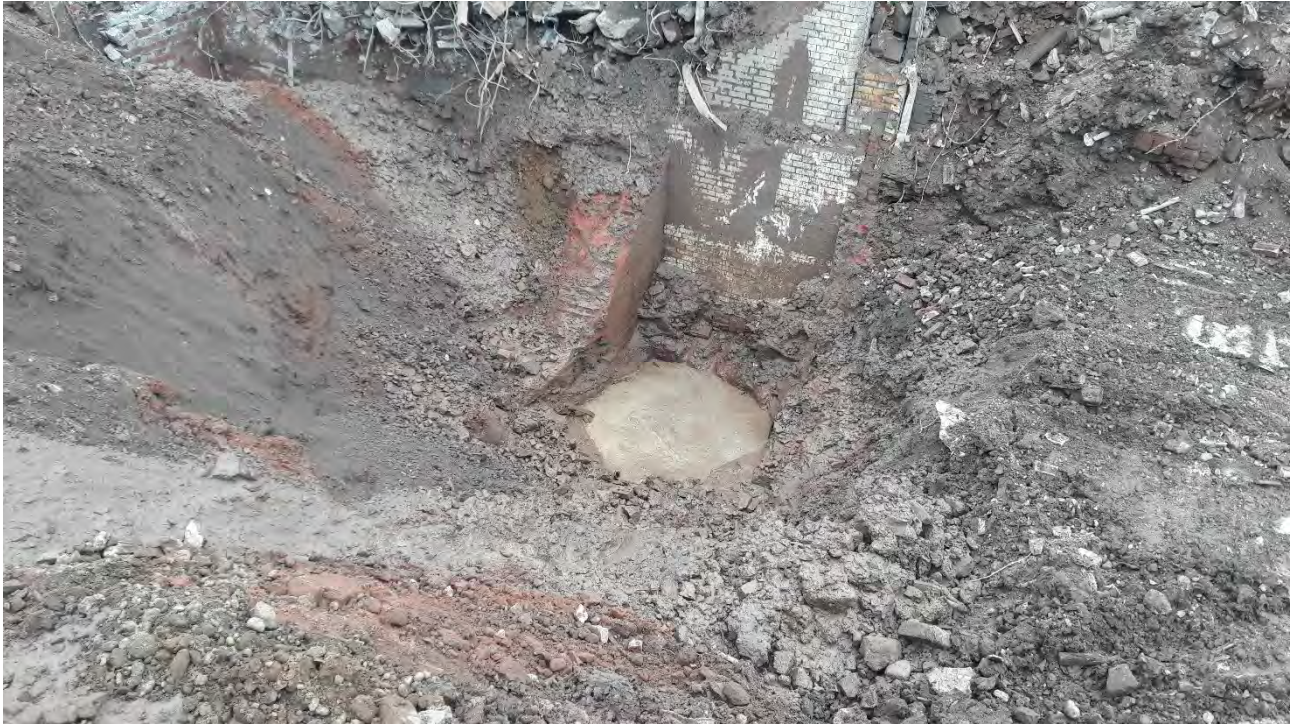
Located on 28/4/2020 at 383831.2E 399206.6N, elevation 23.15mAOD – Approximately 2400mm diameter with no casing.
