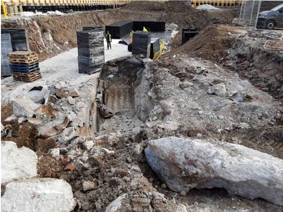
Removal of 2no. USTs. Remains of concrete surround shown in foreground. One tank partially removed and one in-situ.
