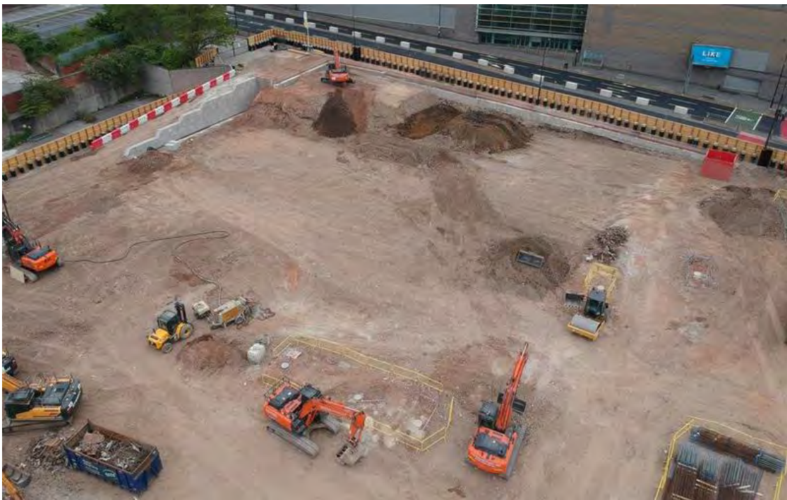
Aerial view showing stockpiles and formation of remediated site levels. Piling operations and materials also shown.
