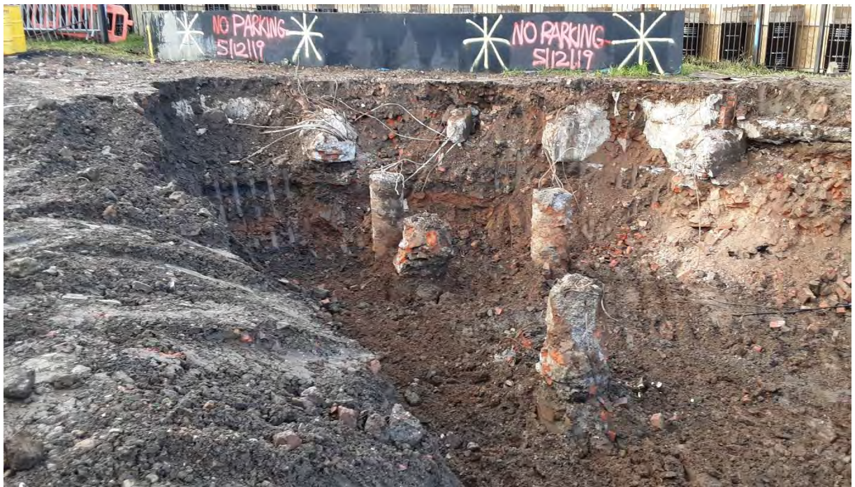
Further examples of relict foundations encountered and subsequently removed during enabling works.
