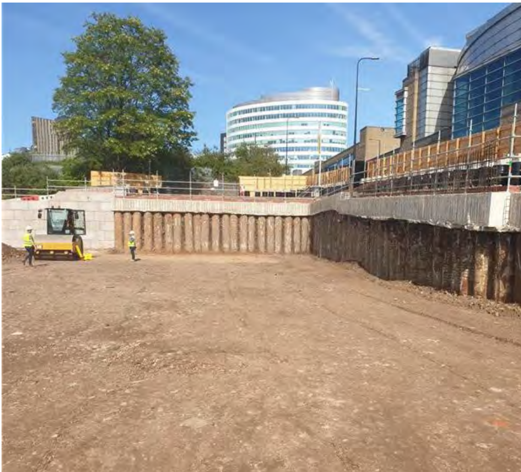
Remediated site levels.
