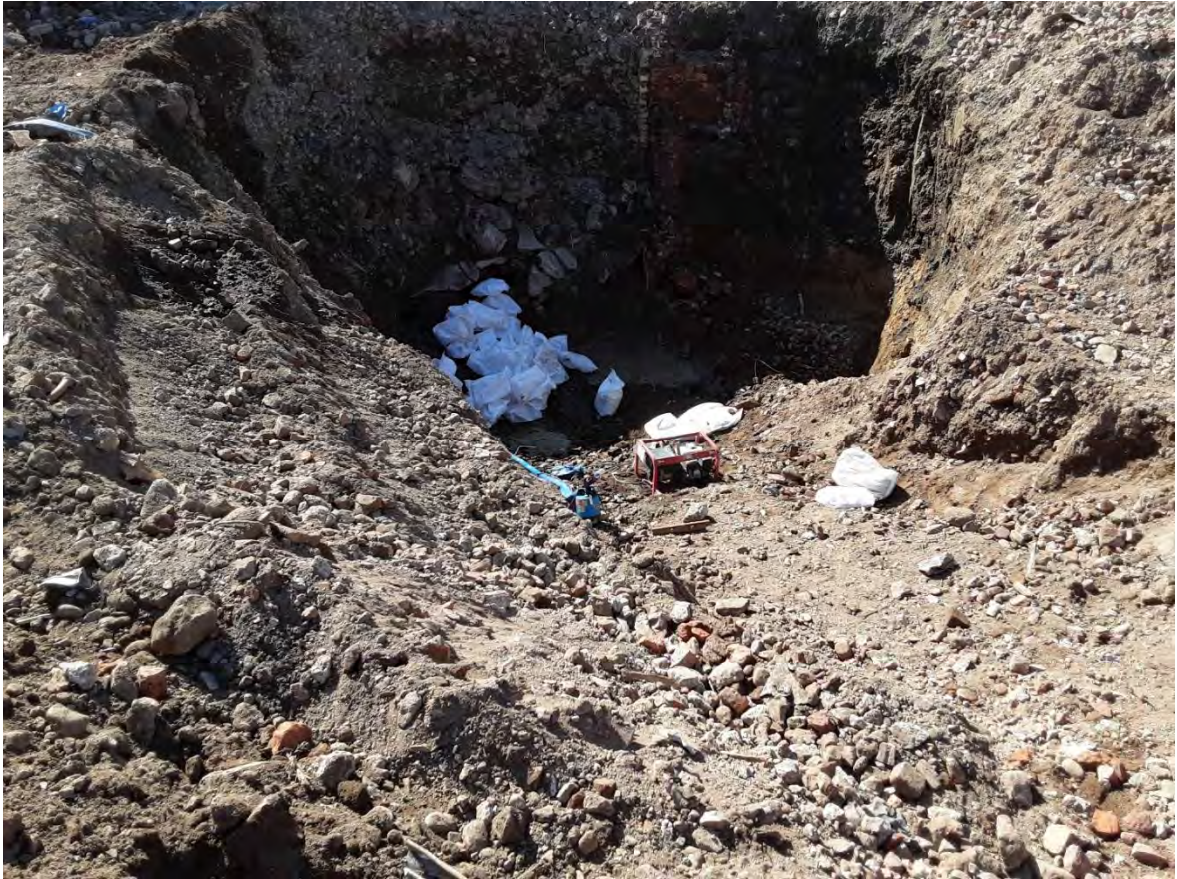
Bentonite seal now installed. Empty bags and retracted pump shown adjacent to abstraction well.
