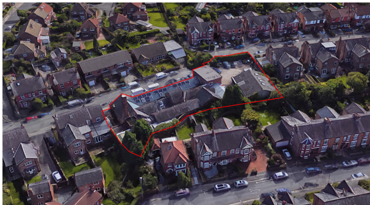
kingsley road site aerial looking east
