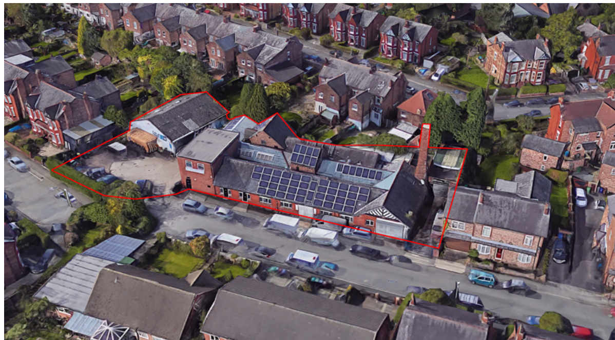
kingsley road site aerial looking west
