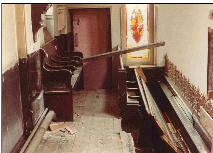
Works to the Ladies Gallery c 1983/4. Raked platform & seating removed.
