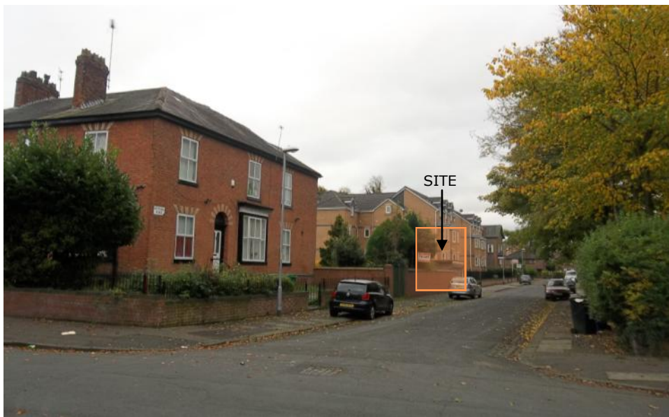
VIEW SOUTHWARDS FROM BROOK ROAD
