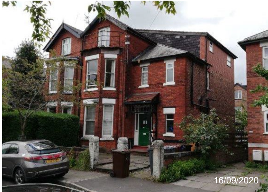
Site photos of 6 Oak Avenue. Chorlton Manchester
