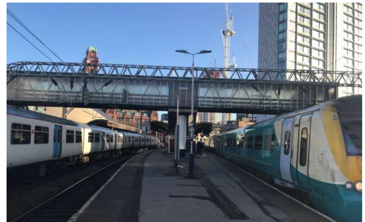
Figure 11: View along the platform of MORS.
