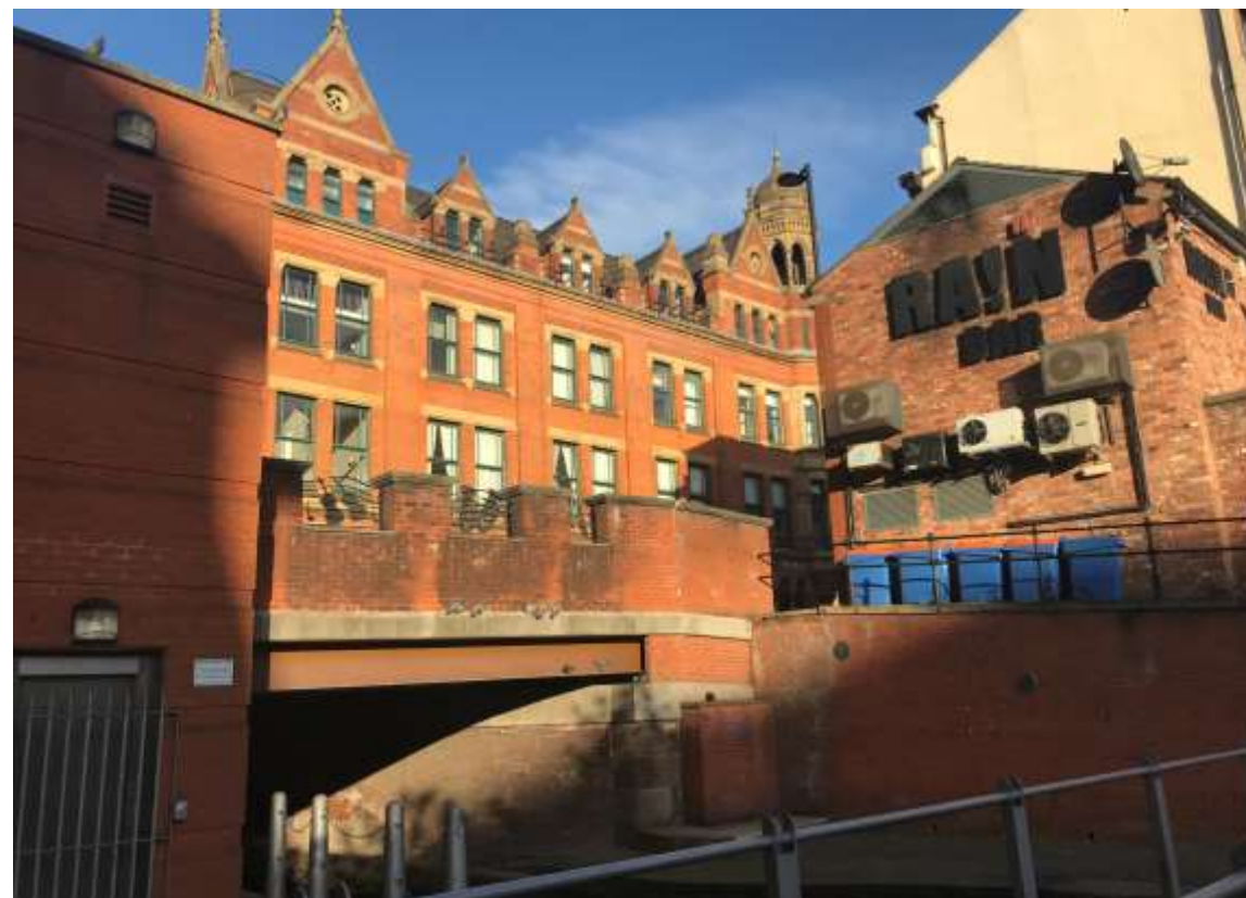
Figure 14: Photograph showing Chepstow House from the lock.
