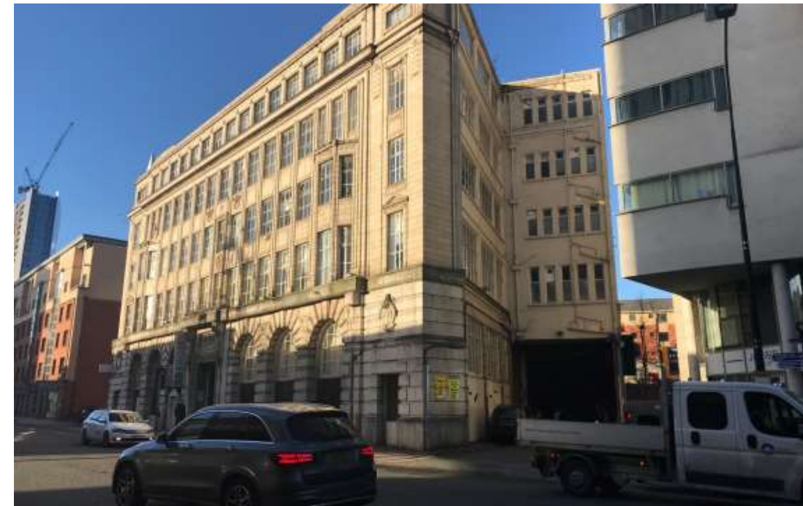
Figure 20: Photograph showing Barclay House viewed from Whitworth Street West, looking west
