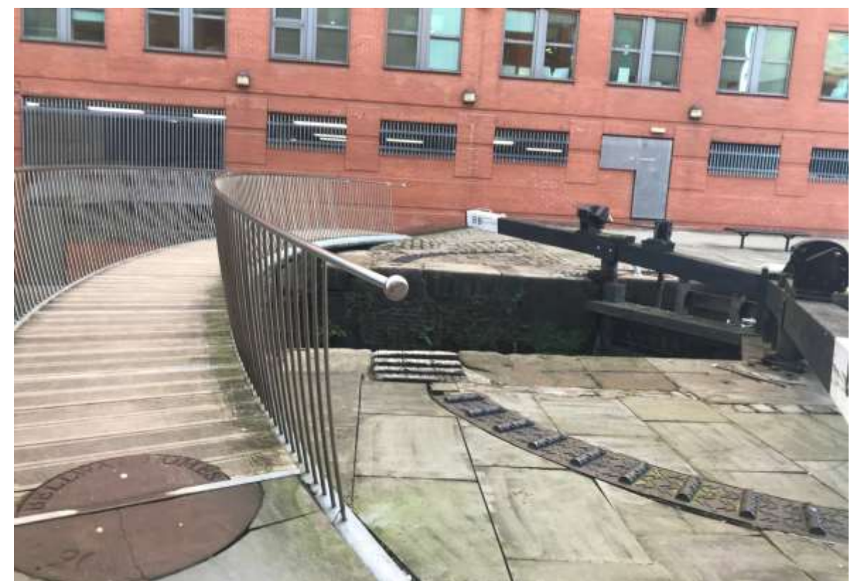
Figure 15: Photograph showing the lock's new pedestrian bridge.
