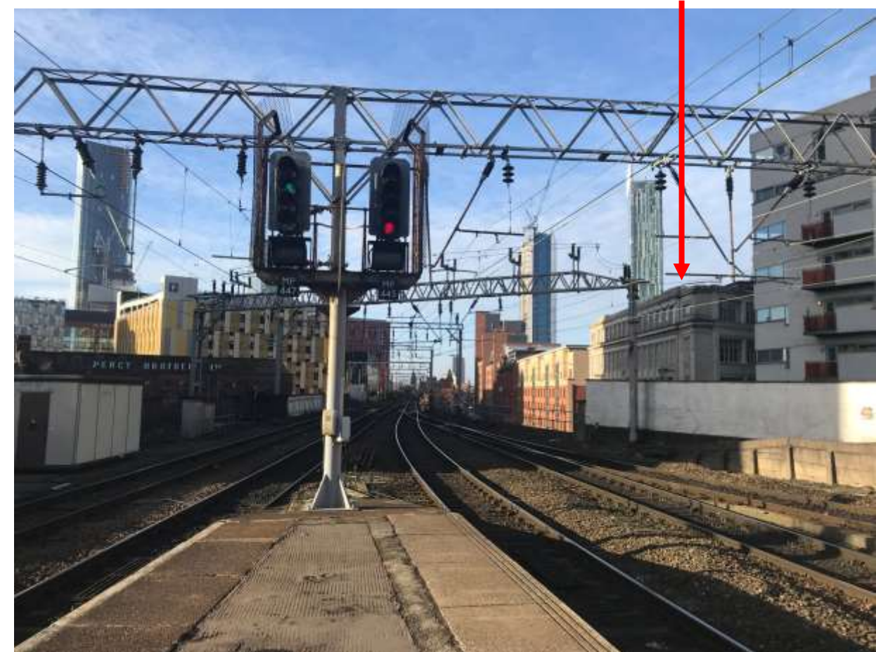
Figure 2: Photograph showing Barclay House from the far end of the platform of Manchester Oxford Road Station (MORS), looking west.
