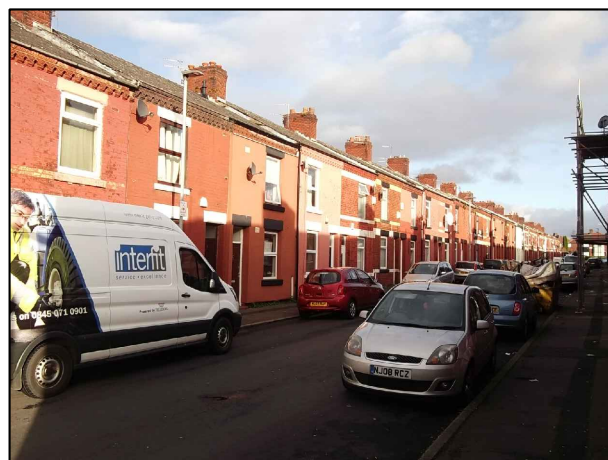
29. Madison Street, typical long terrace off Vine Street
