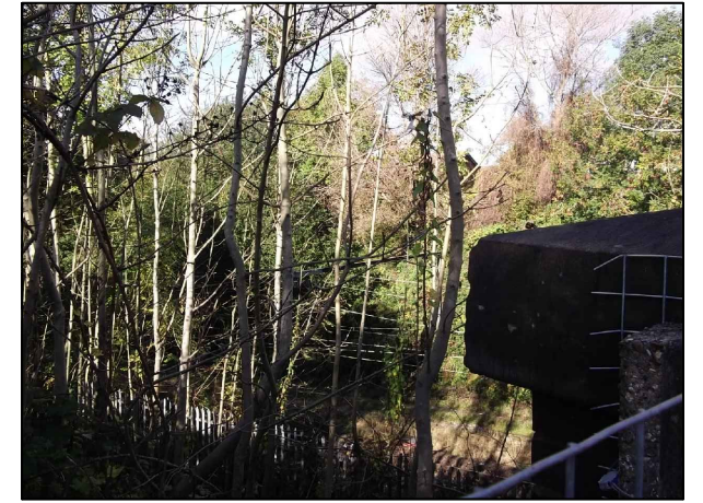
23. Railway from bridge
