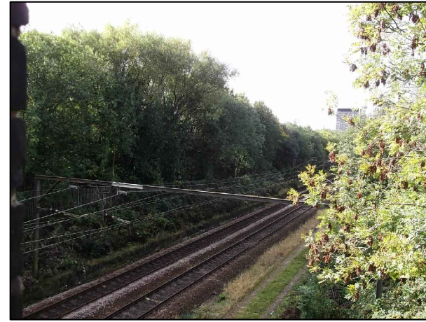
22. Railway looking west
