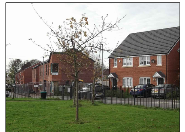
31. Infill development Gathurst Street
