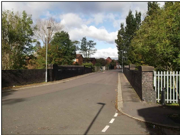
40. Vine St bridge
