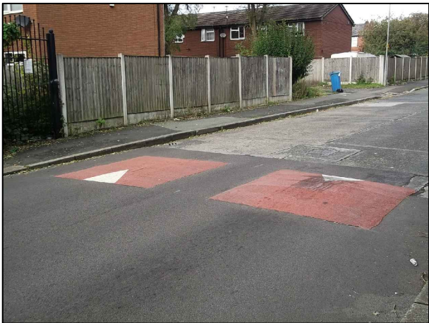
41. Traffic calming north of Vine Street bridge
