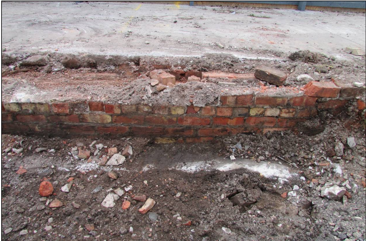
Plate 8: View of wall 202 looking south-west. The remains of the concrete floor can be seen in front of the brick wall
