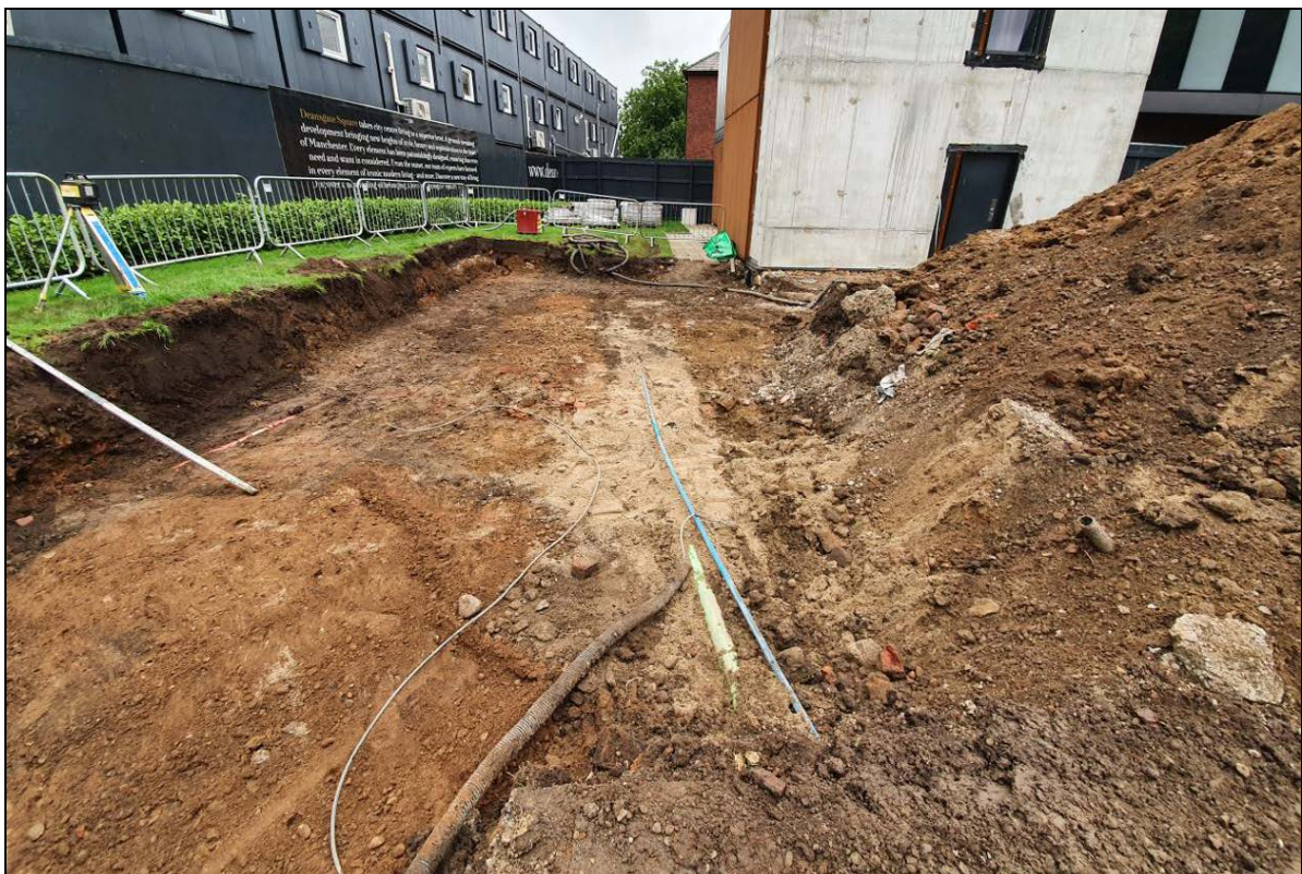
Plate 24: The second area fully excavated
