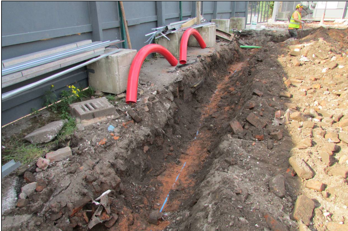
Plate 20: View along the excavated service trench (Area 3)
