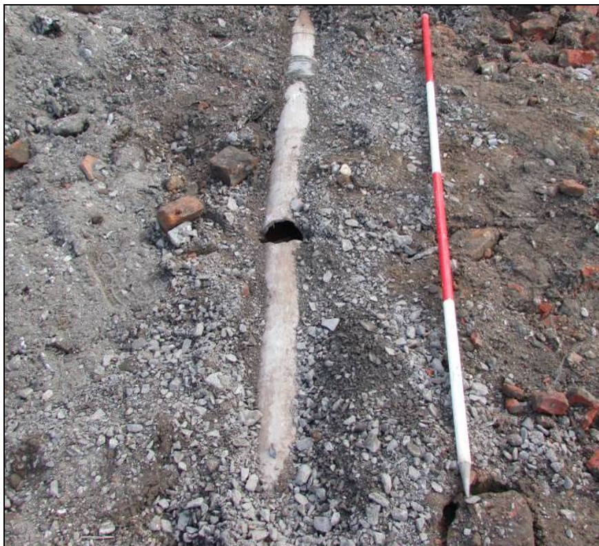
Plate 17: Modern ceramic pipe cutting across Area 2
