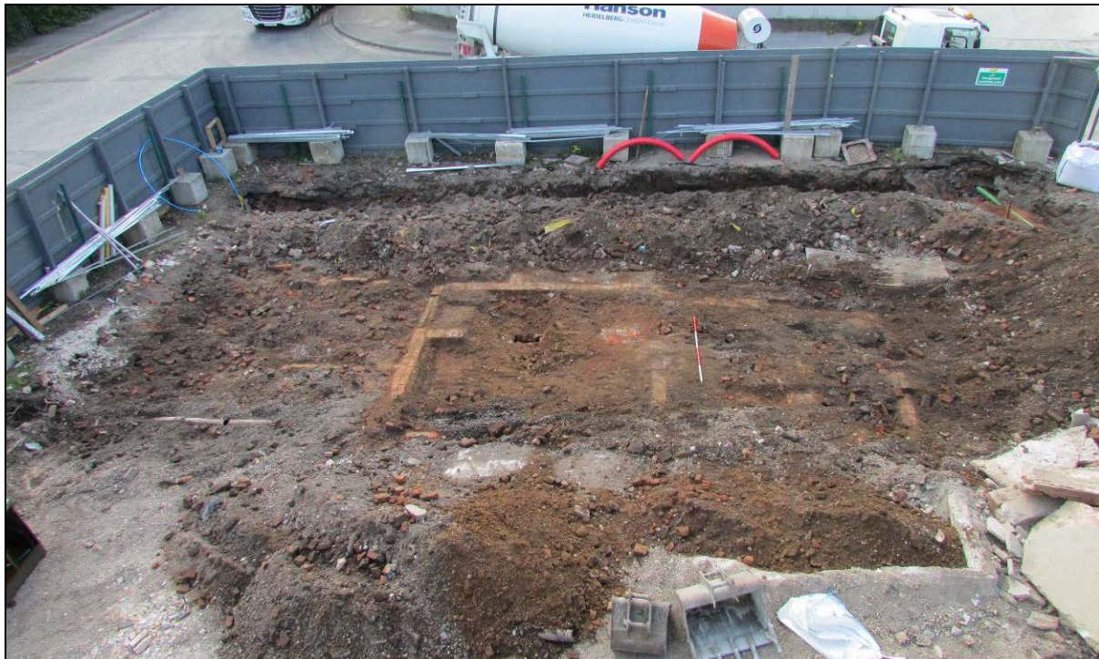
Plate 15: General view of Area 2, with service trench (Area 3) in the background, looking south-east
