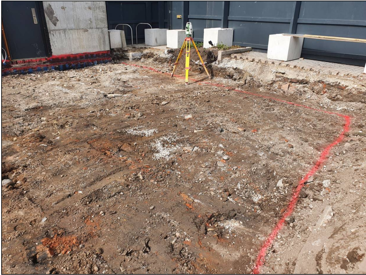
Plate 22: View across the area to the south of the 2018 building, showing the 20 th -century demolition material, overlying the natural geology
