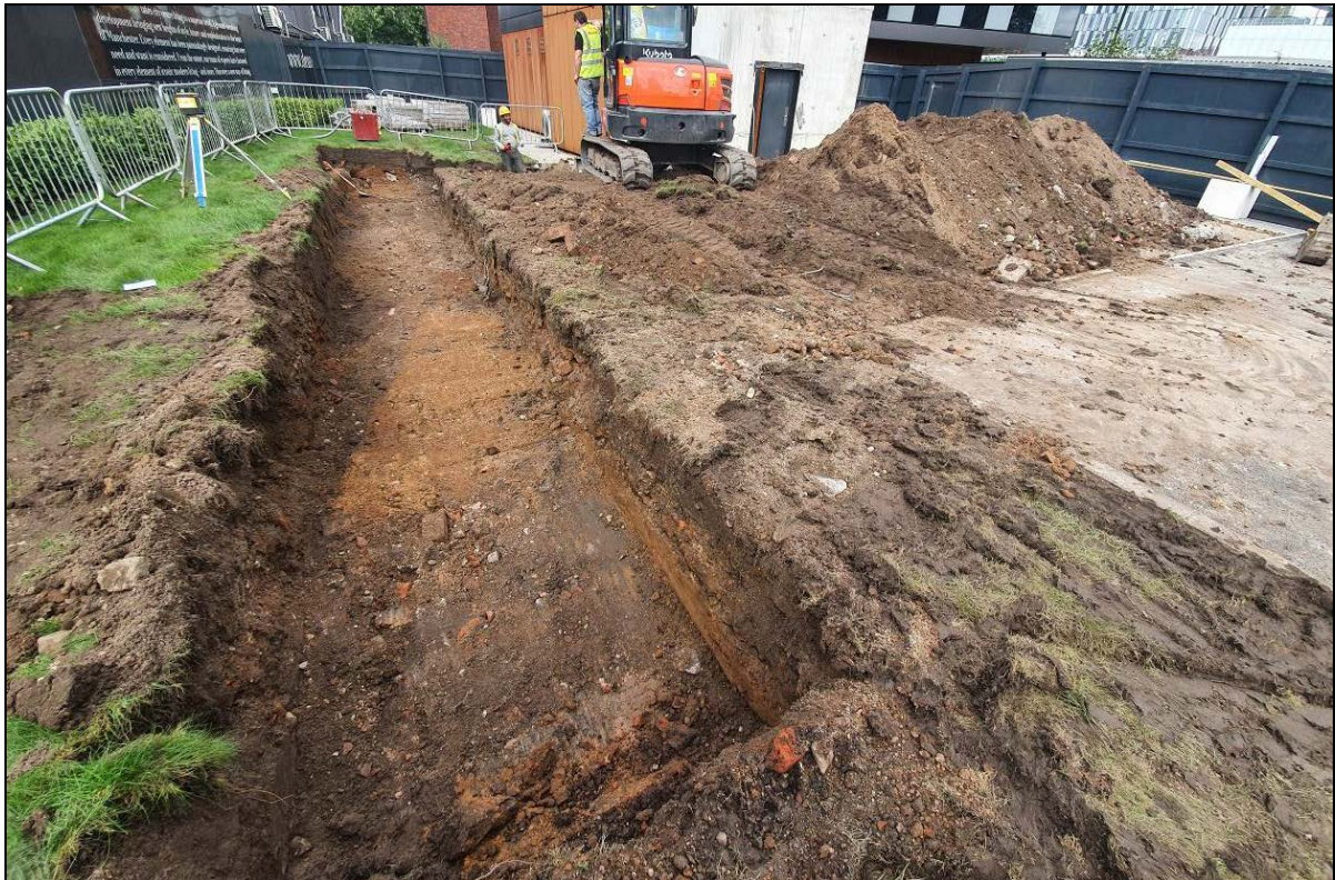
Plate 23: Trench excavated along the western side of the 2018 building, showing a modern service trench cut into the natural drift geology, and vestiges of modern mixed demolition material overlying the natural geology
