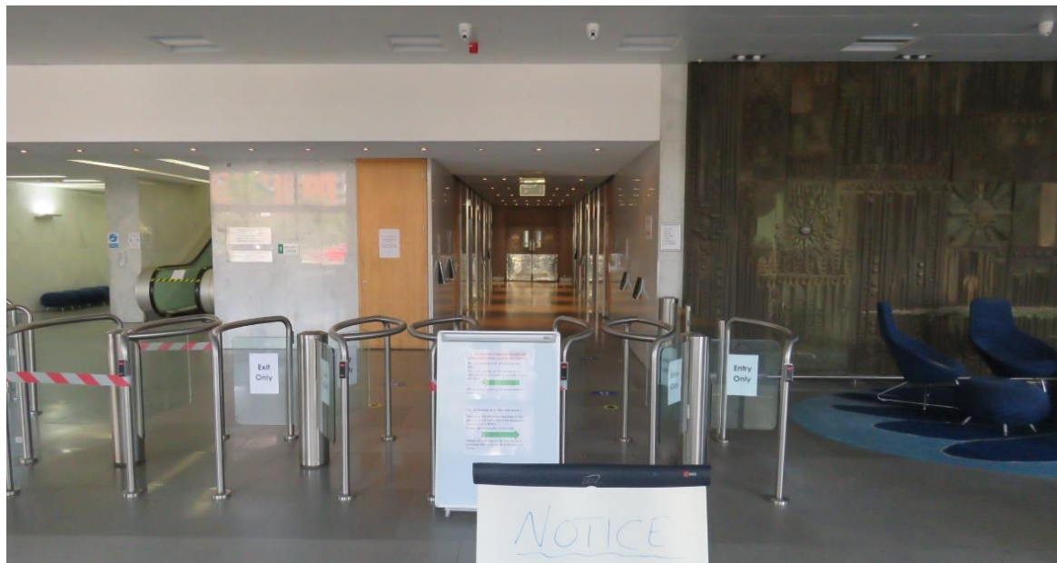
00-01 Looking south from the revolving doors, showing the security gates and the William Mitchell mural.
