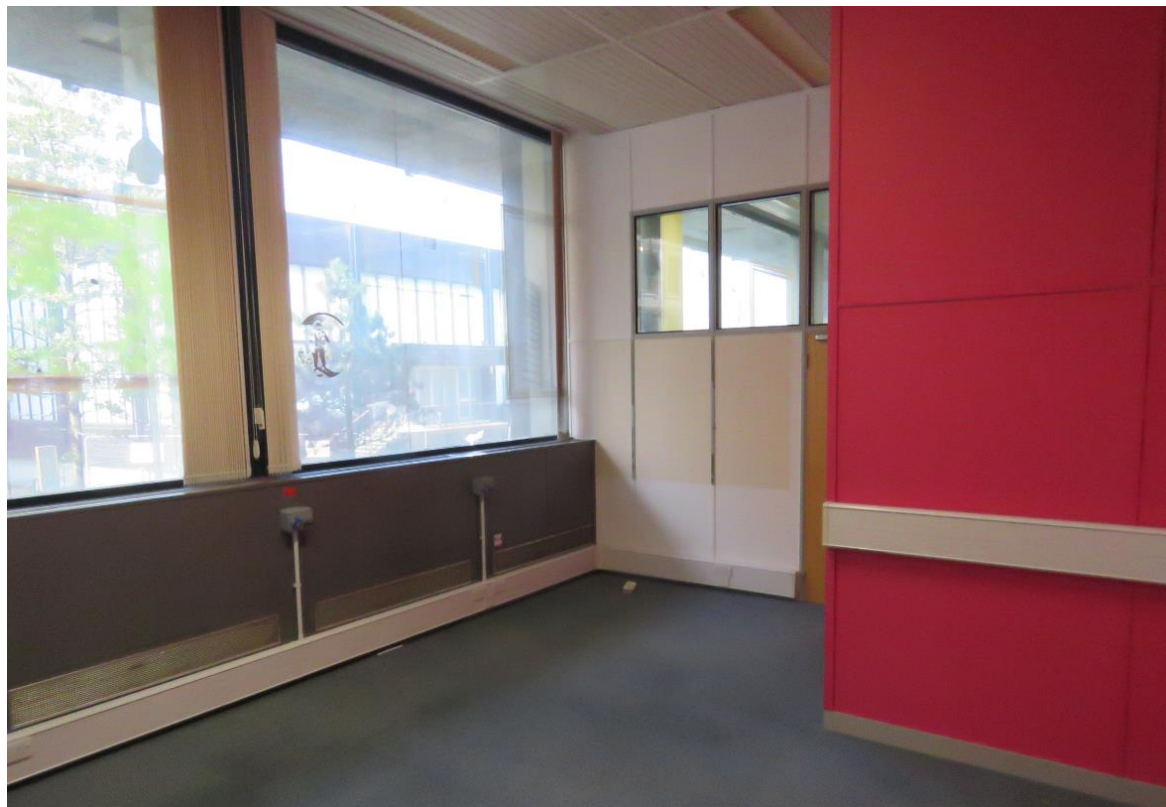
00-11 Looking north-west within an inserted former post-room office.
