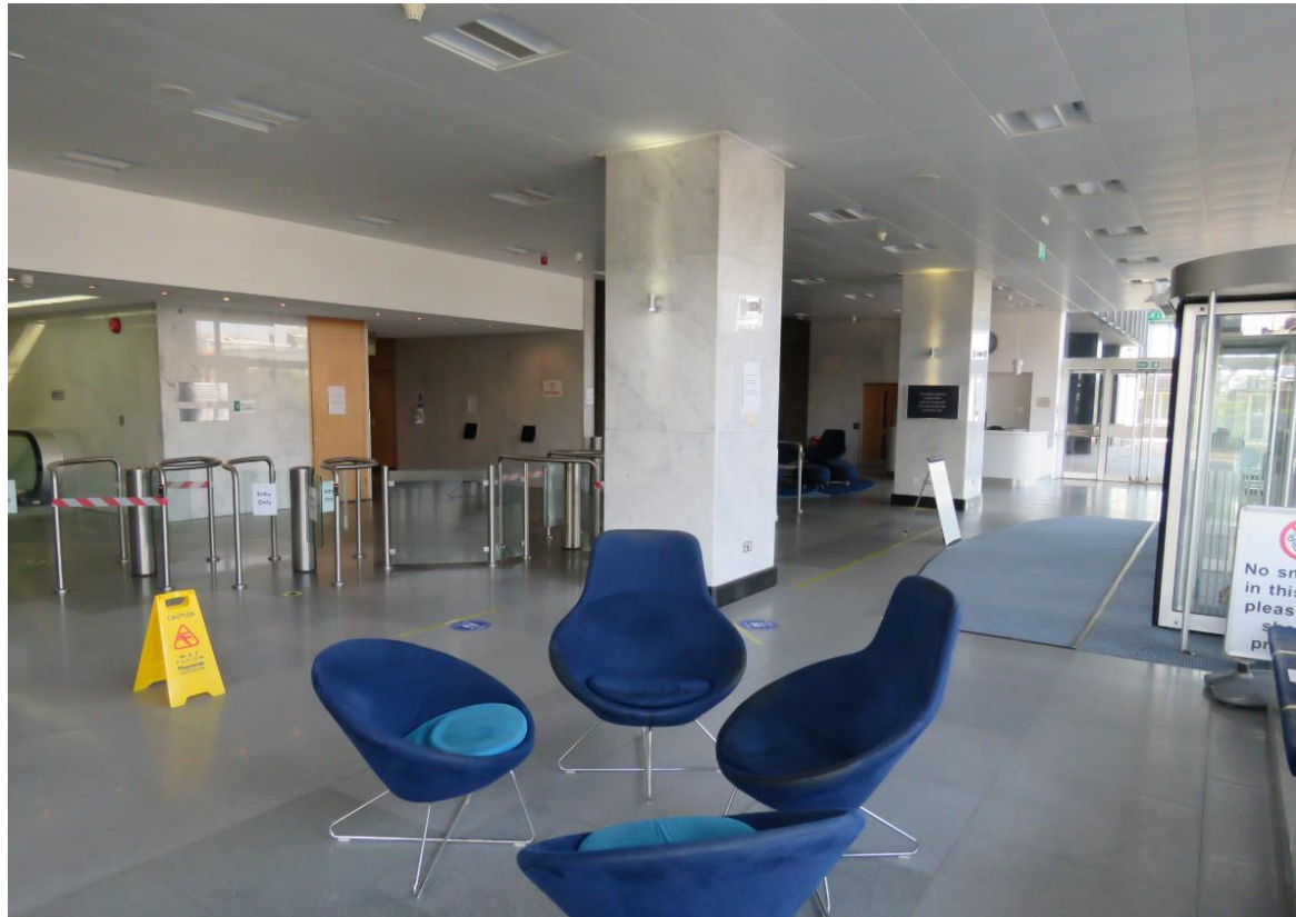
00-04 Looking south-west across the reception hall showing the inserted ceiling and column cladding.
