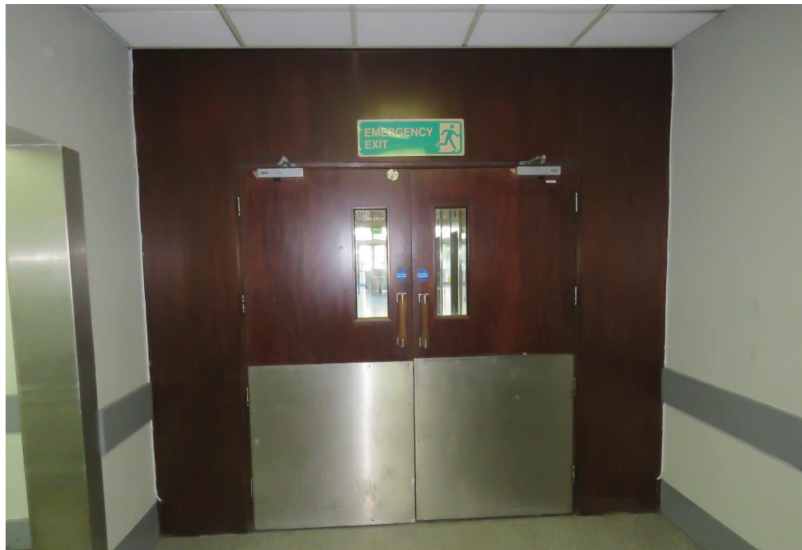
00-21 Looking north toward the original doors to the lift lobby.
