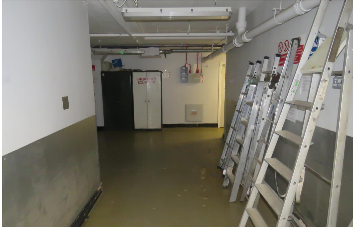
00-24 Looking south into the service area.
