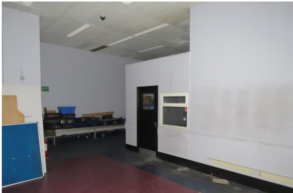
00-13 Looking north-east towards the Tel lift terminus in the post room.
