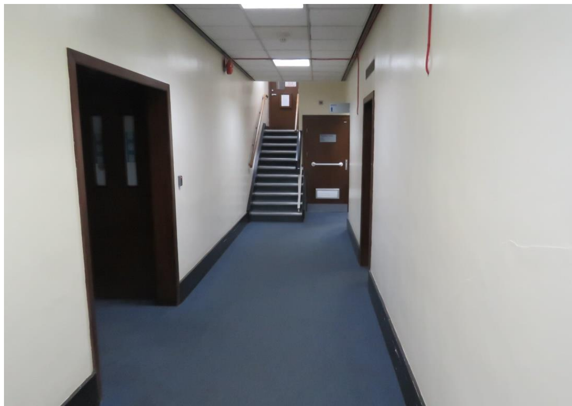
00-29 Looking south along the access corridor and stair to the mezzanine care-park.
