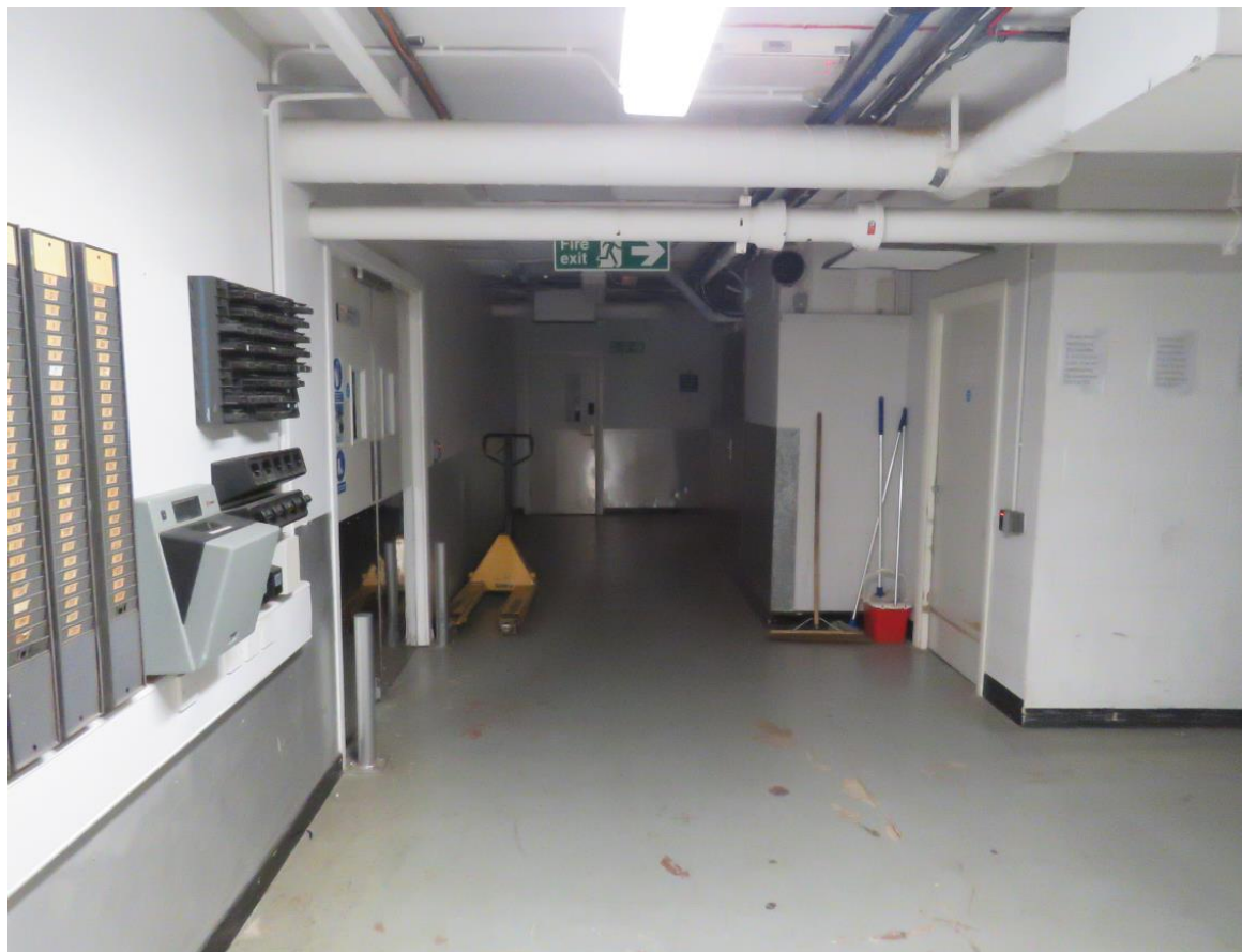
00-25 Looking east along the service corridor.
