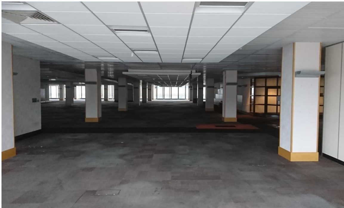
02-41 Looking west across the podium office floor from the Riga Street elevation.
