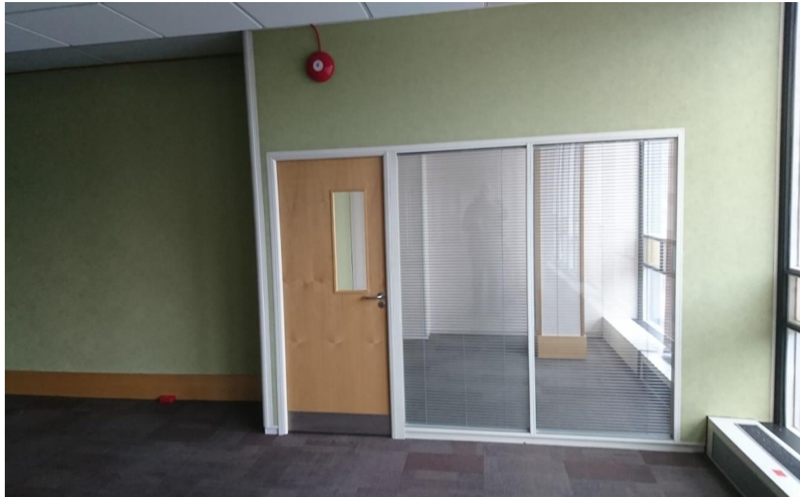
02-32 Details of inserted south-east office partition.
