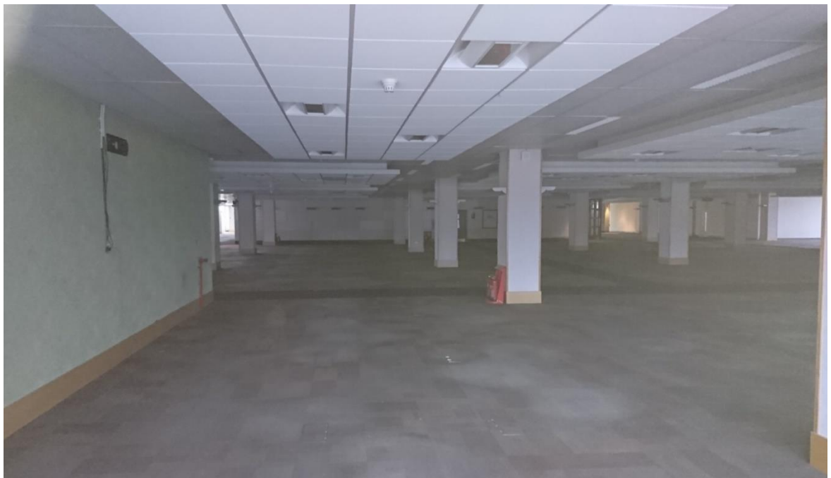
02-31 Looking north across the podium towards the central core and lift lobby.
