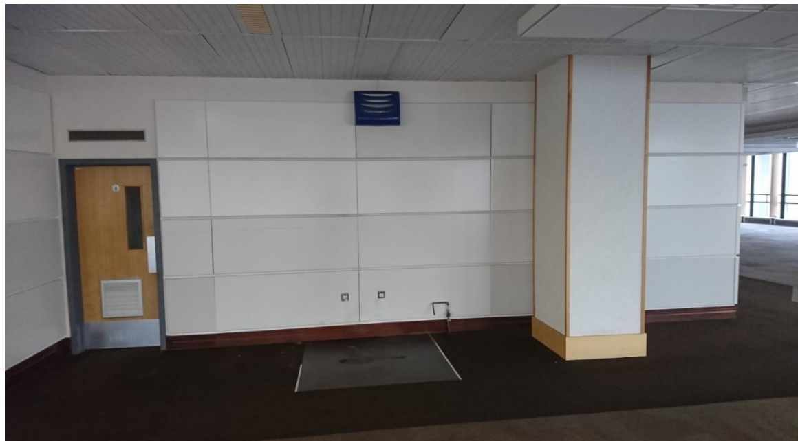
02-13 Looking south at the replacement partitions enclosing the toilet block.
