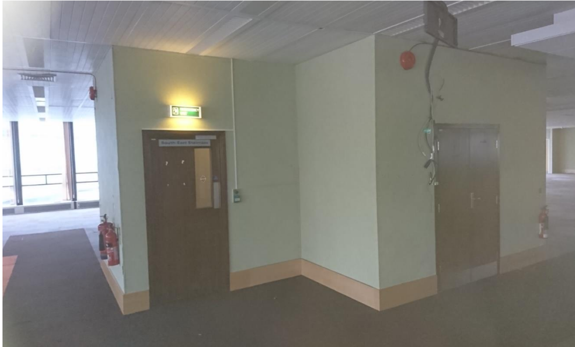
02-34 The enclosure to the south-east stairs.
