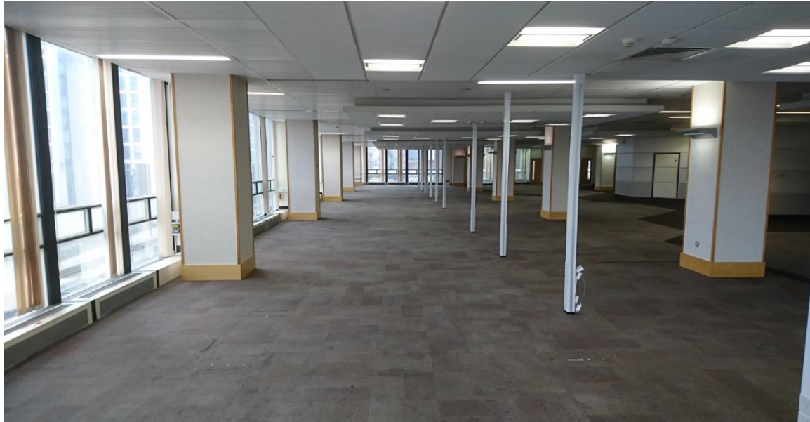
02.06 Looking east across the tower office floor, showing replacement ceiling and floor covering.
