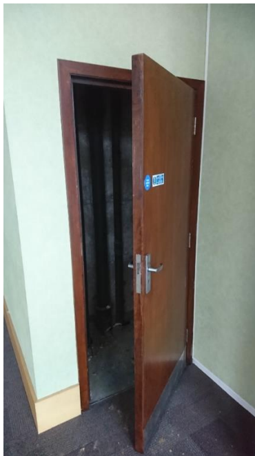
02-27 Plant room door.
