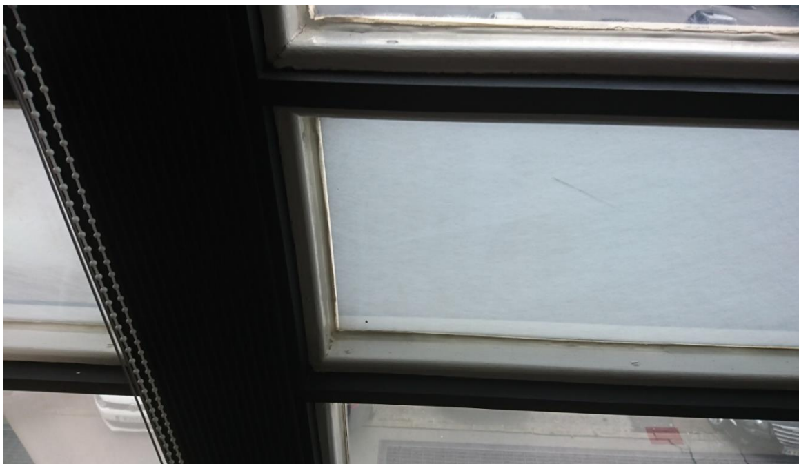
02-39 Details of the beading and glazing to the windows on the podium.
