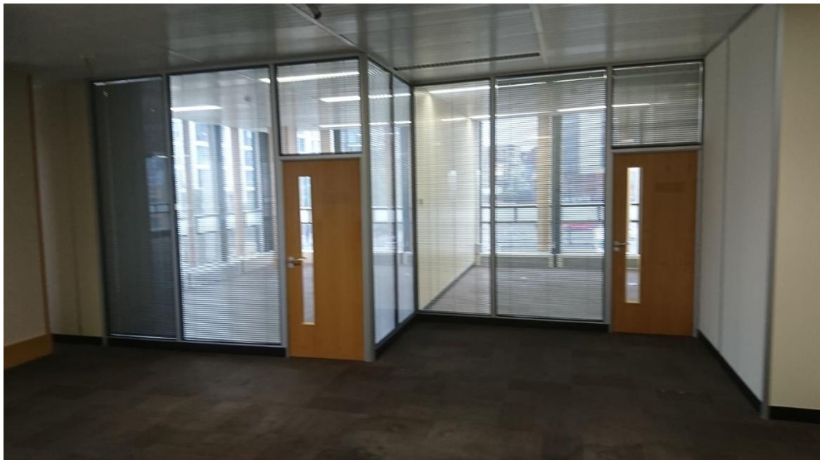
02-47 Looking east through the inserted north-east corner offices in the tower office.
