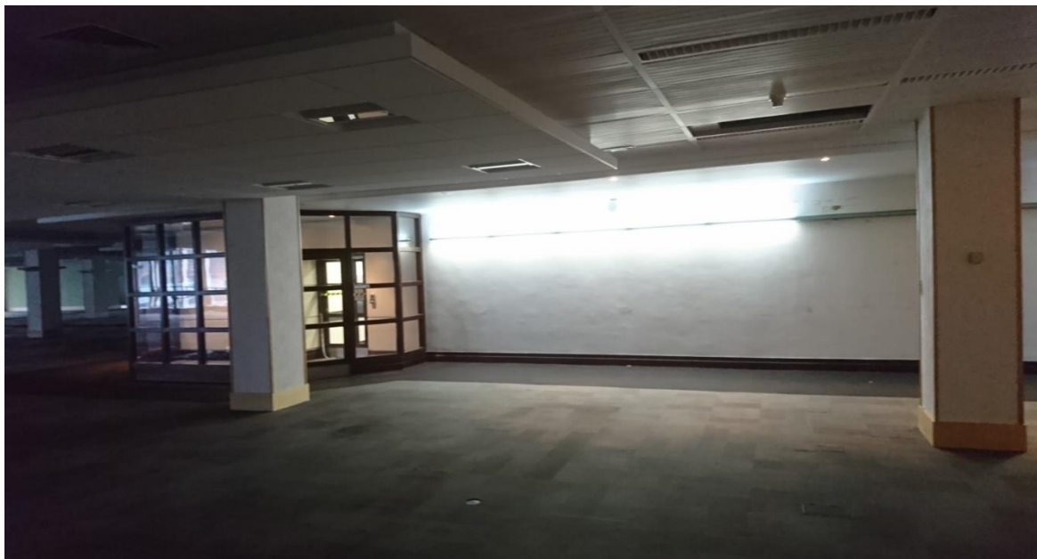
02-45 Looking west across the podium/tower office junction to the escalators enclosure.
