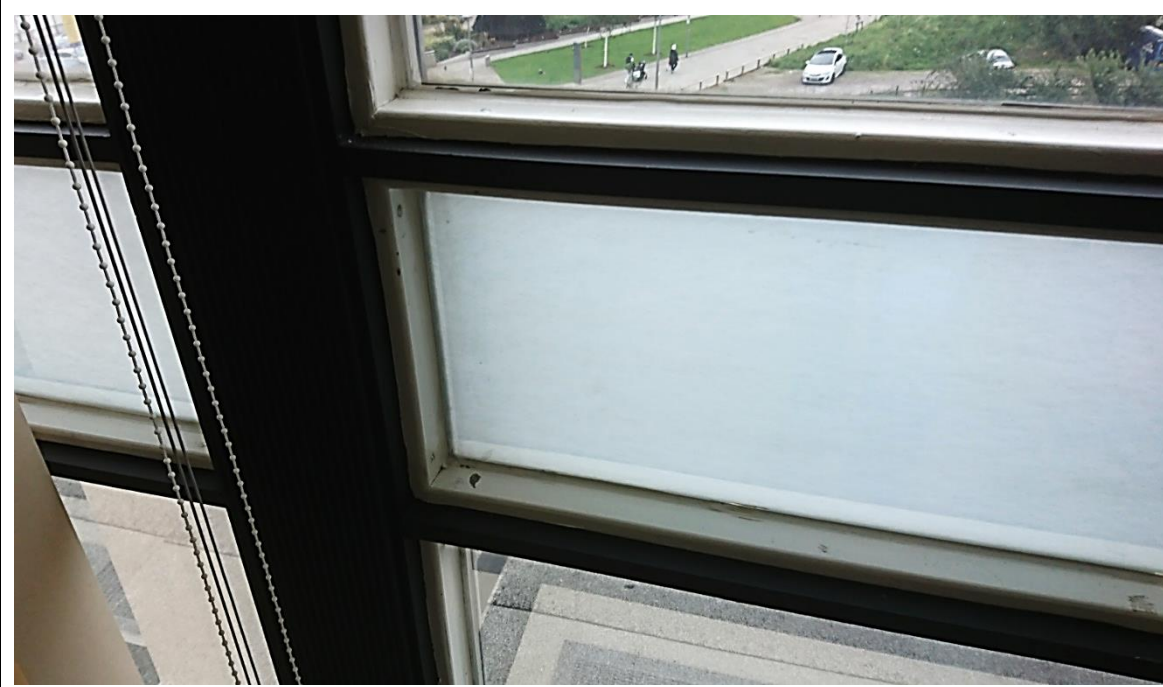
02-08 The timber beading to the north-elevation windows, showing the encased fibre-glass/asbestos which creates the opaque glazing panels.
