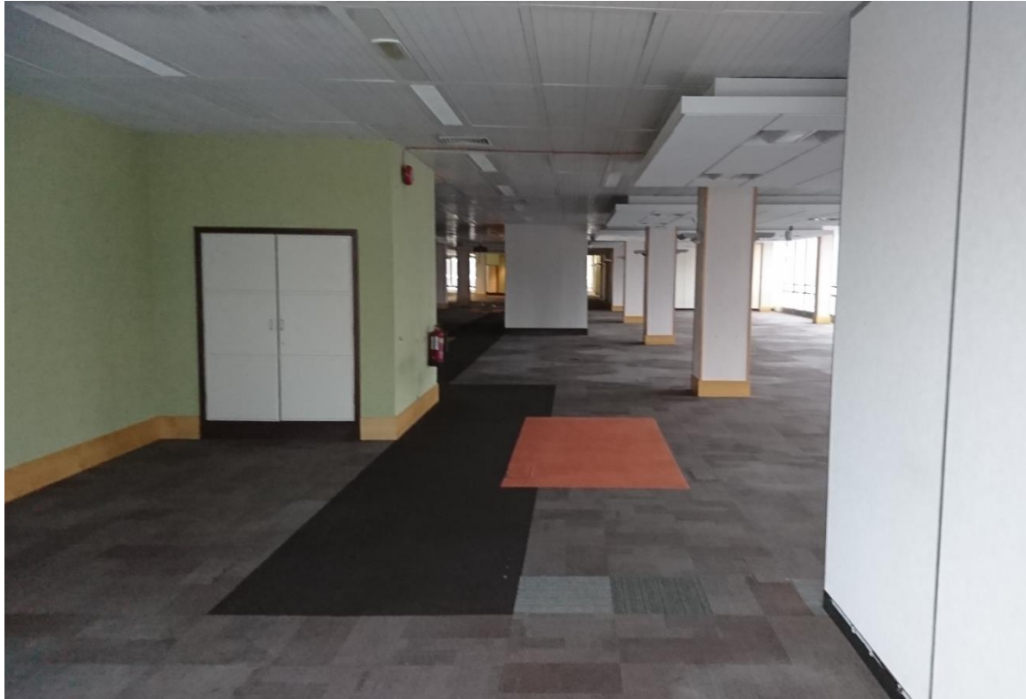
02-36 Looking north from the Hanover Street elevation, showing the south-east stairs to the left.
