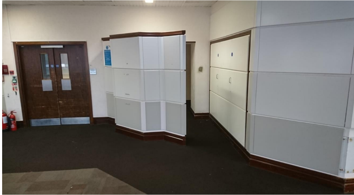
02-10 Looking south toward the entrance and the non-original screens which enclose the Telelift document transportation system (see also Section 4.3 above).
