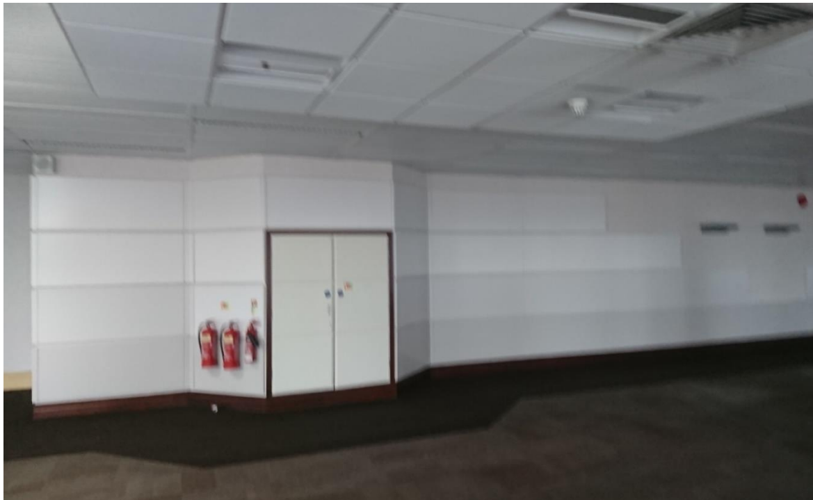
02-15 Example of the replacement partitions, ceilings and interior wall décor.
