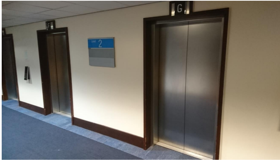
02-02 Detail of the lift cars and timber surrounds.
