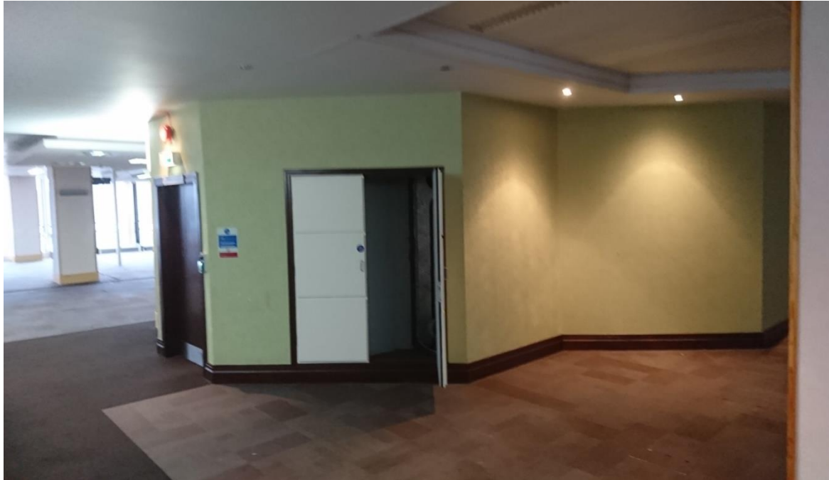
02-46 The enclosure of the inserted, north-east escape stairs.
