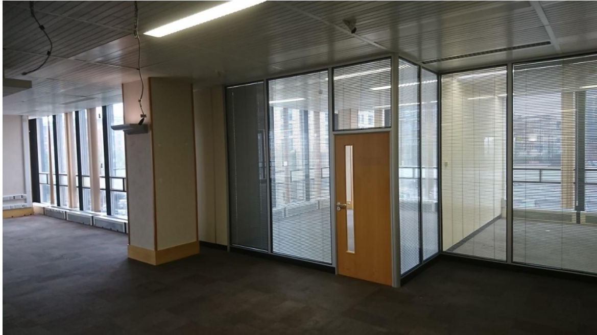
02-48 The inserted north-east corner offices in the tower office.
