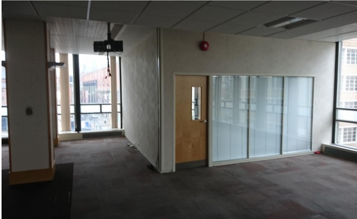
02-22 Inserted south-west corner office within the podium office floor.
