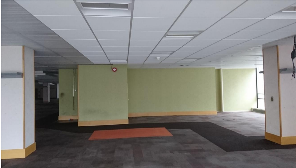
02-24 Looking north toward the inserted enclosure of the north-east stairs.
