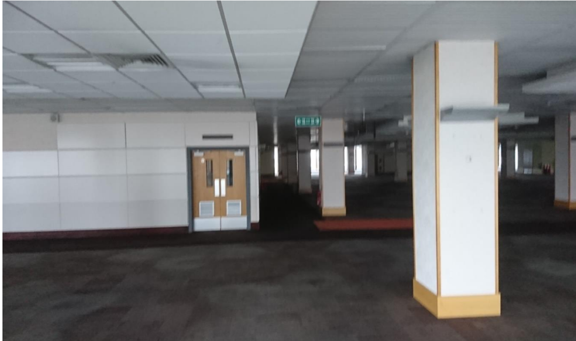
02-16 Looking east across the junction between the tower and podium.
