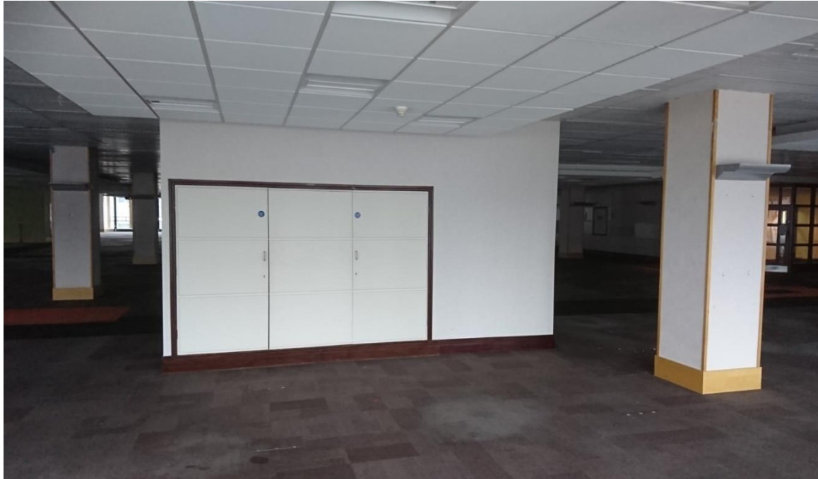
02-40 Inserted IT plant room in the podium.
