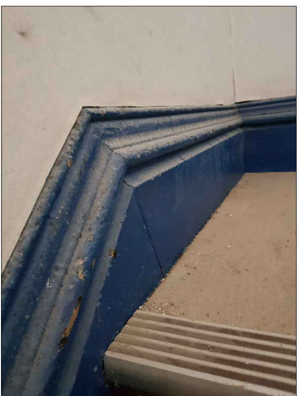
Typical Skirting Board secondary staircase / landing
