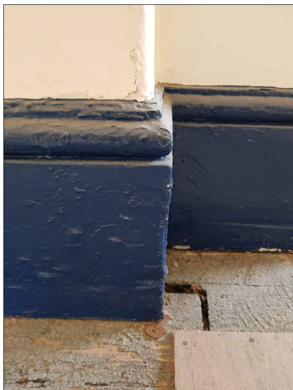
Typical Skirting Board to 2nd floor rooms and hall
