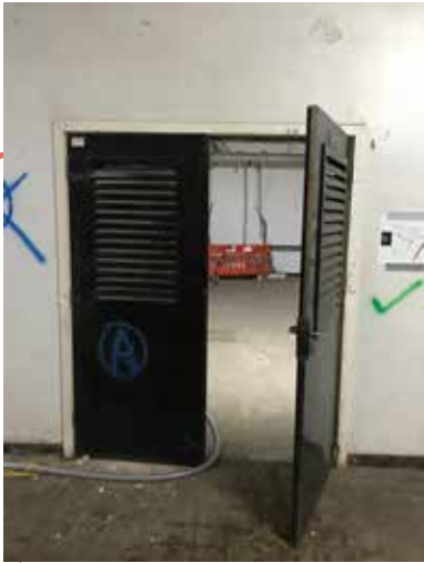
Louvred door from B'' corridor to propose storage space
