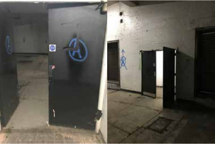
Fire door into proposed storage space
