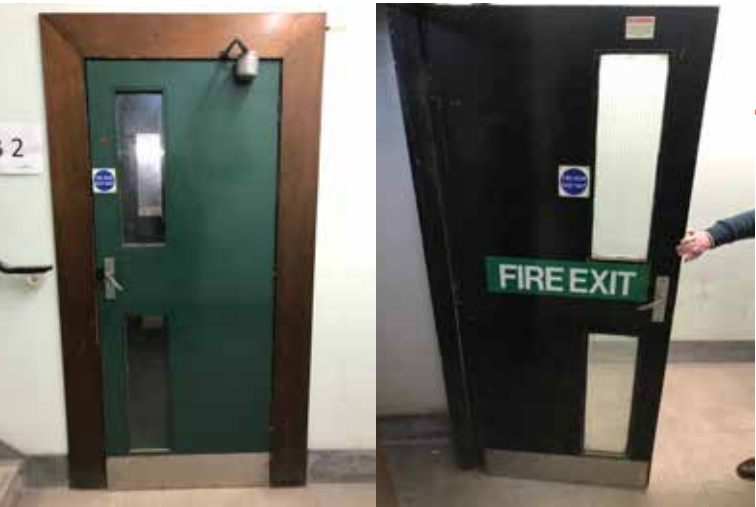
Fire door from stair core to lobby
