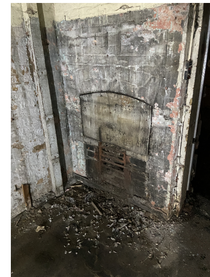
PHOTO SHOWING THE CURRENT CONDITIONS OF THE FIREPLACE AND CAST IRON FITTINGS
