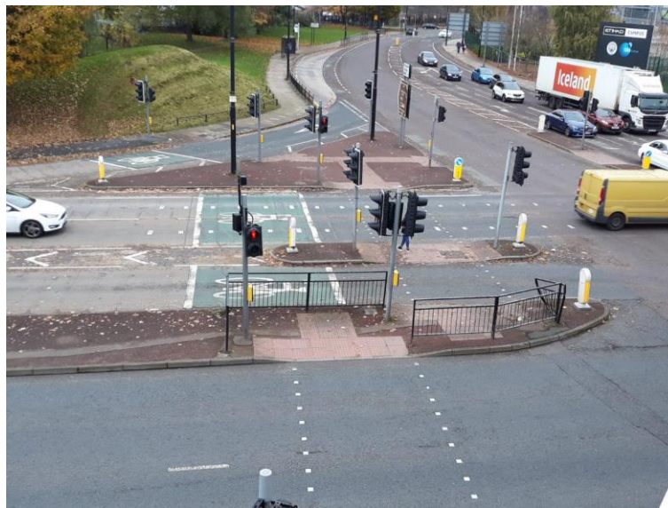
Photo 4: Advanced Stop Line (ASL) at the Alan Turing Way/Ashton New Road Junction
