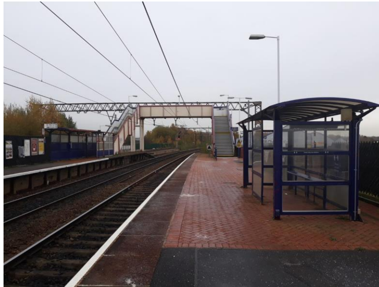
Photo 7: Ashburys Rail Station
