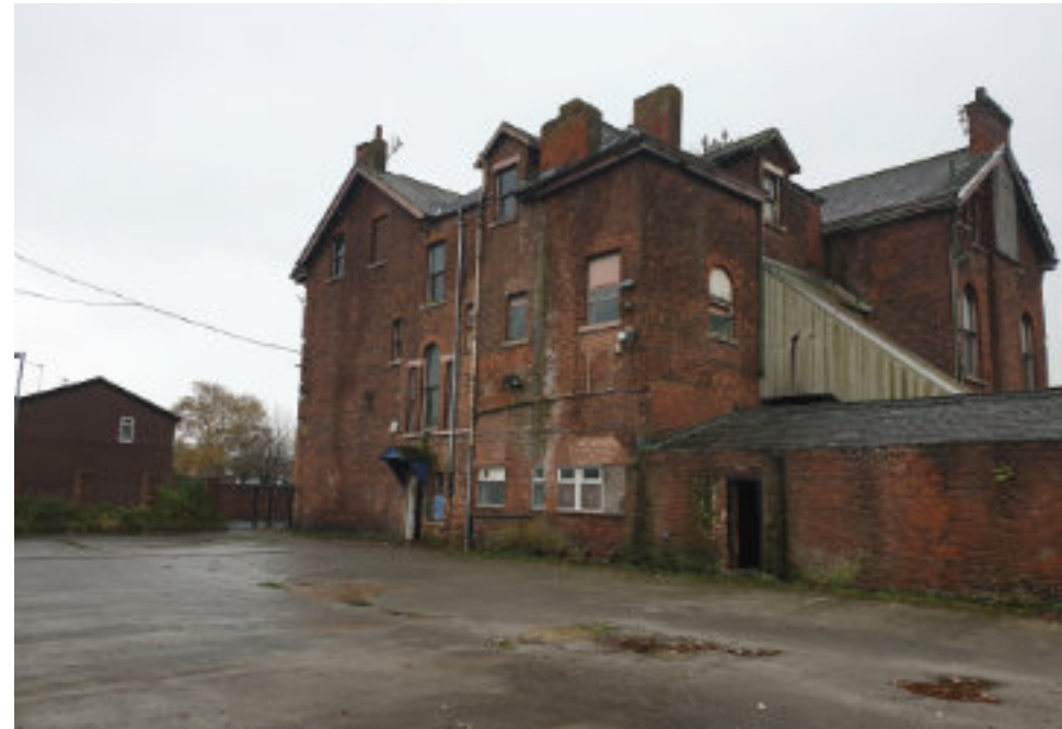
View from car park looking East
