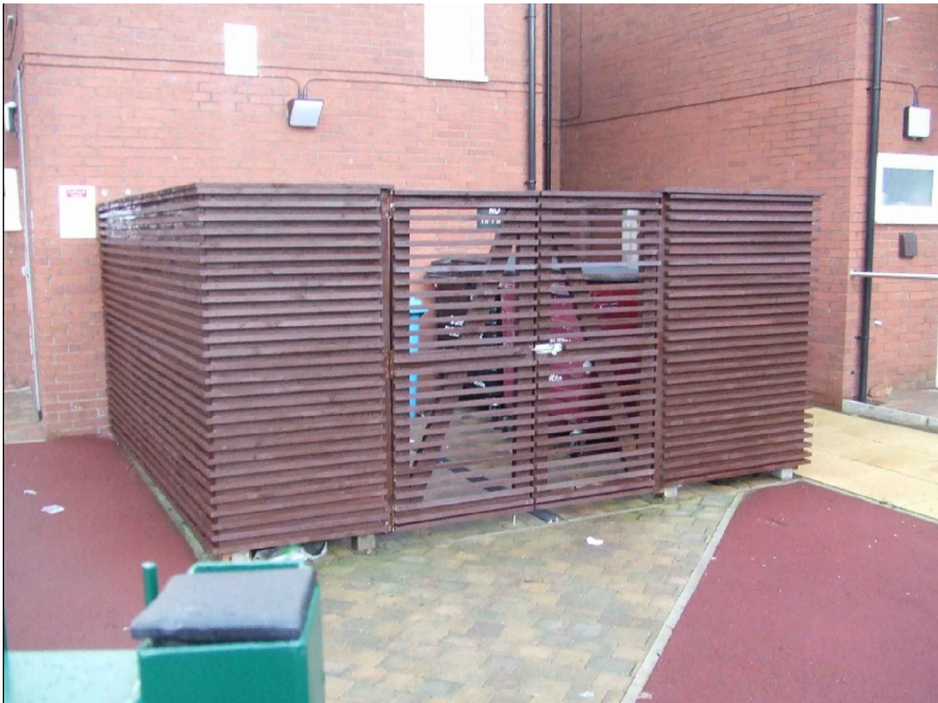
New Bin Storage
