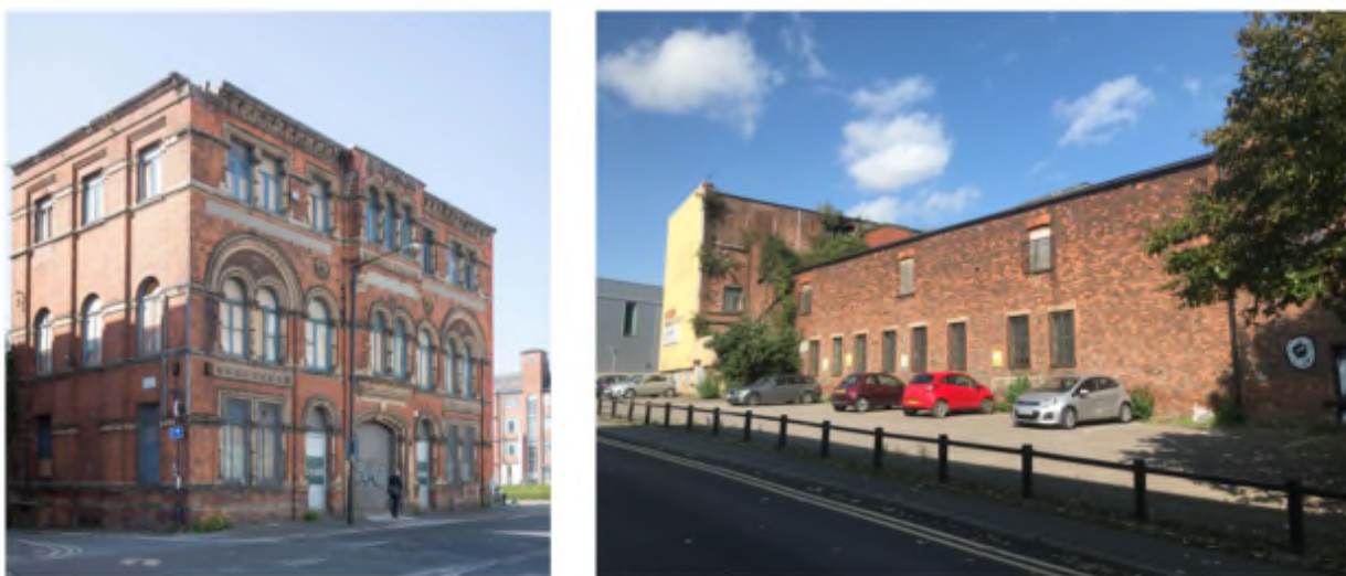
Figure 3.1 Photographs of the Site, left being the decorative frontage of the showroom, and the right image showing the original outrigger (Source: OMI, 2020)
