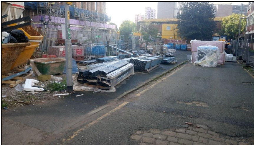
Photograph 3 showing an area of bare ground/building materials and equipment
