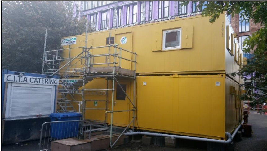
Photograph 6 showing some of the portable cabins on site
