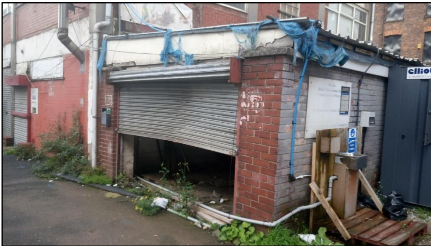
Photograph 10 showing the eastern extension on the three-storey building
