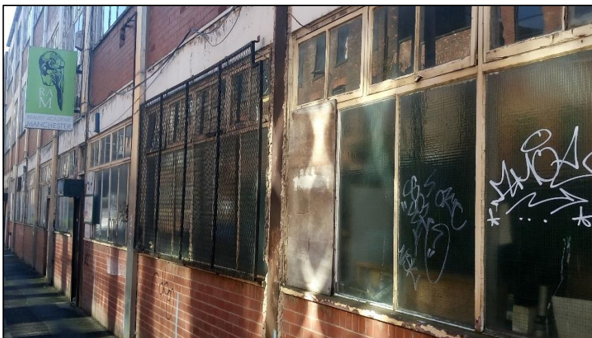
Photograph 9 showing some of the windows across the building
