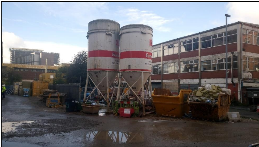
Photograph 7 showing the silos on site
