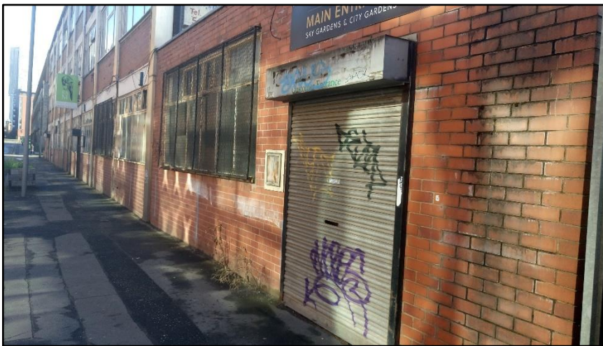
Photograph 8 showing the exterior of the building
