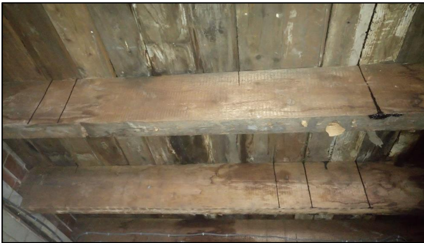
Photograph 14 showing the underside of the roof
