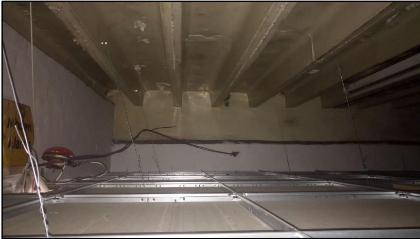
Photograph 13 showing one of the small void spaces between the suspended ceiling and the underside of the roof
