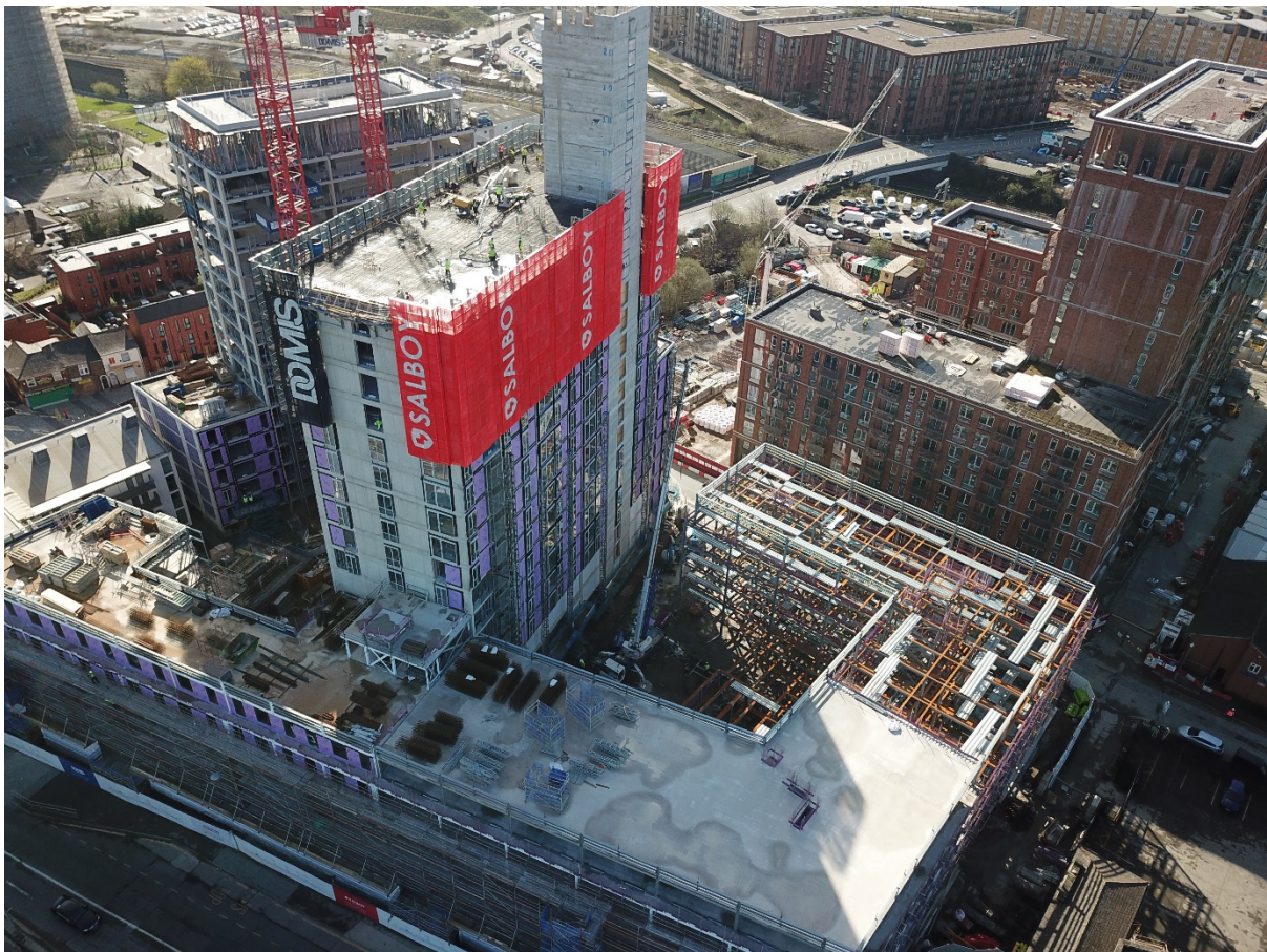
Image of sliding frame safety screens from Crescent project
