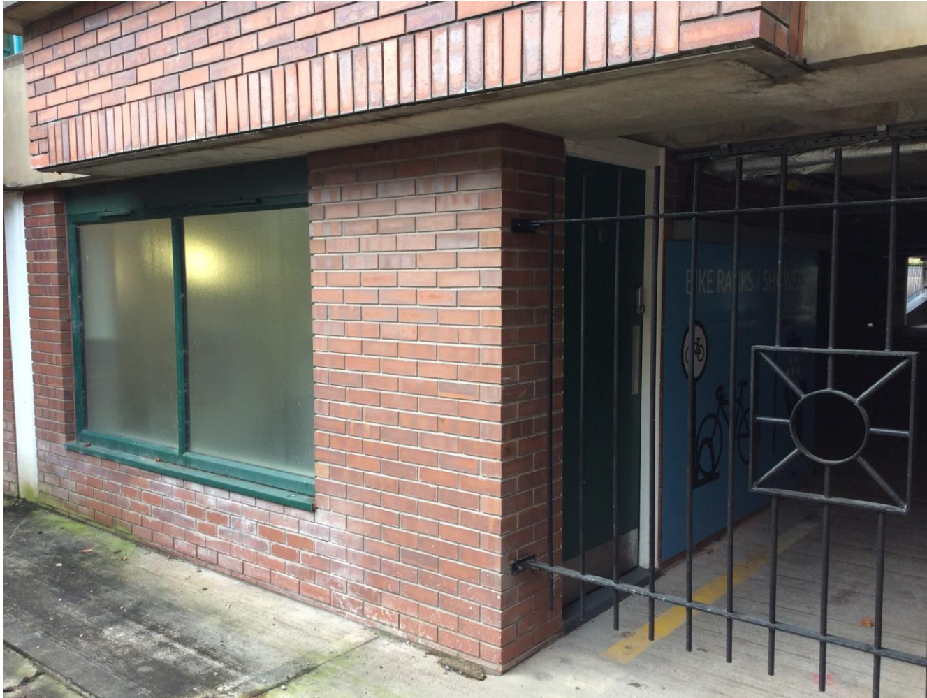
External elevation of the existing amenity block. Basement, Ocean House, Towers Business Park
